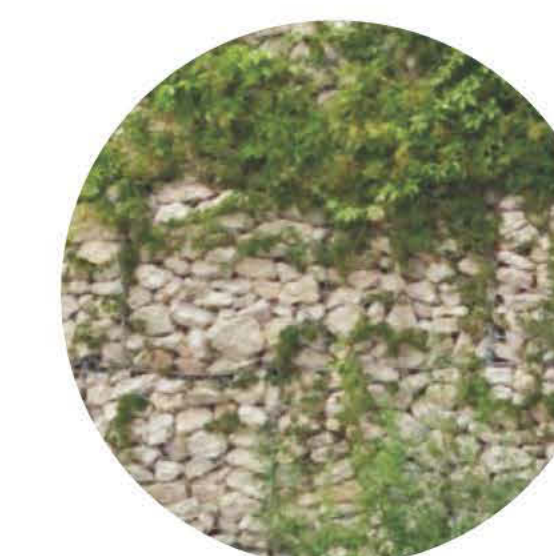
Gabion as foundation for plantlife
