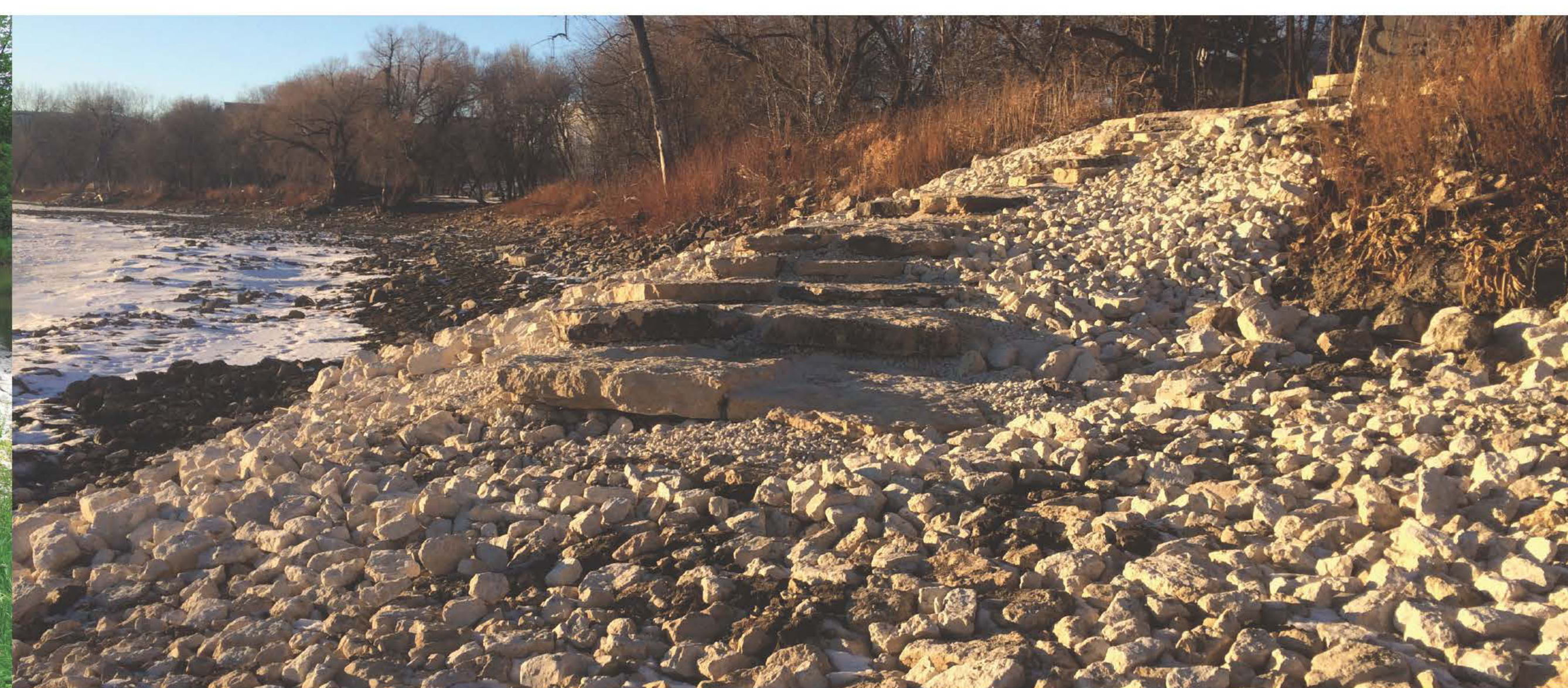
Limestone blocks for fishing and canoe/kayak launch
