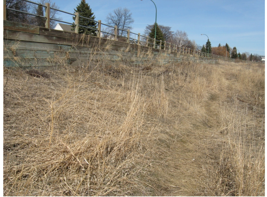
Existing Timber Retaining Wall
