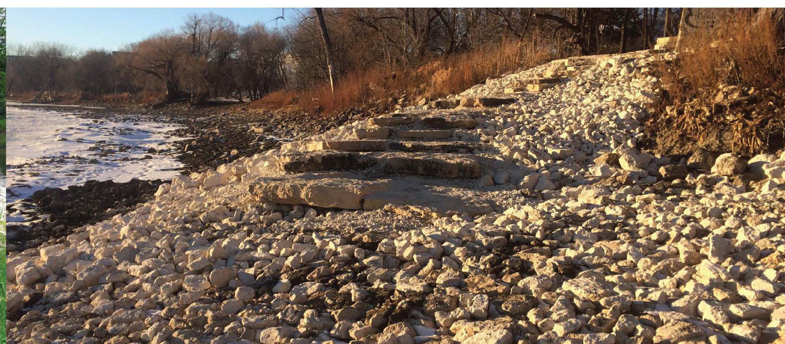
Limestone blocks for fishing and canoe/kayak launch
