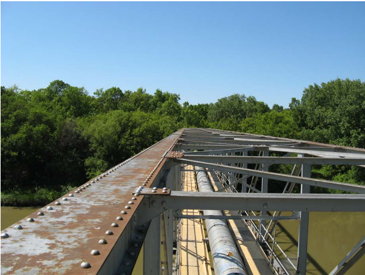
A3-06 - Top of Bridge East Half.JPG
