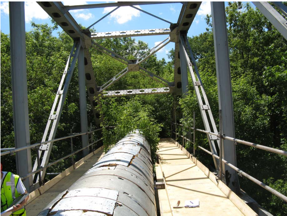
A3-09 - Pipe Insulation and Cladding-South End.JPG
