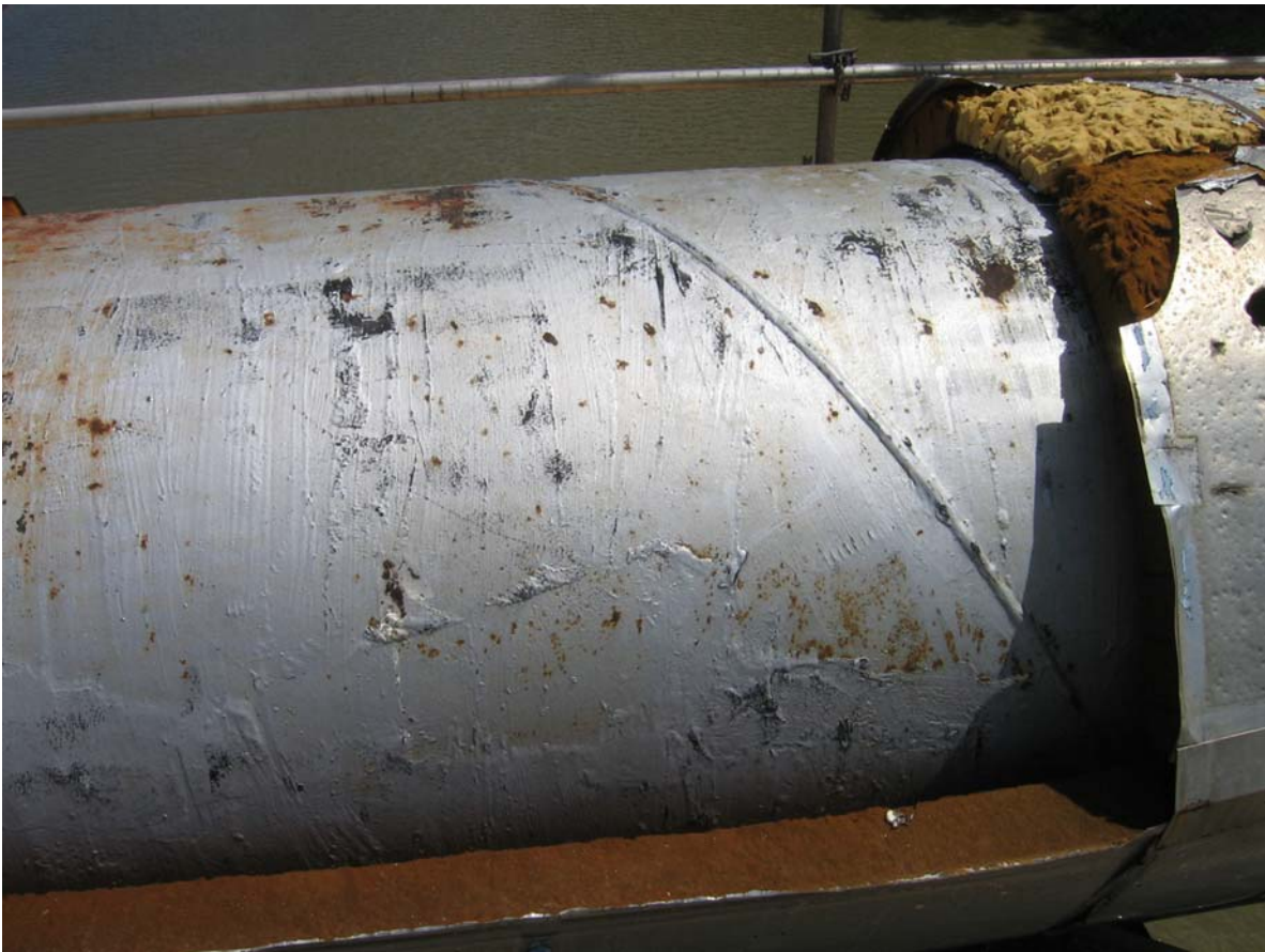
A3-12 - Existing Pipe Coating.jpg
