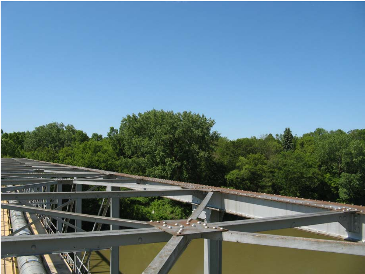
A3-07 - Top of Bridge West half.JPG
