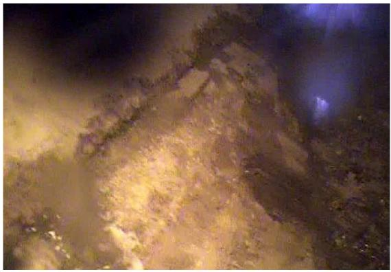
Crack at 9:00 extending from 14m to 16m where large pile of soil was observed. Coincides with the sinkhole at surface.
