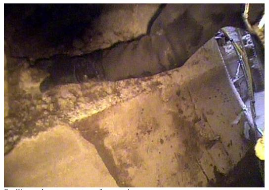
Spalling and past concrete surface repairs
