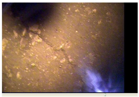
Longitudinal crack along pipe at 12:00 running throughout length or concrete section
