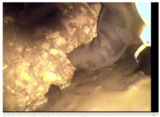
Hole in pipe 11.5 m d/s from chamber at 4:30
