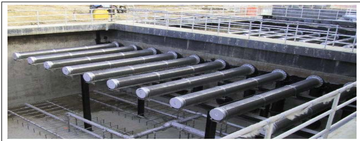
Figure 9.7: Typical Media Retention Screen Assembly
