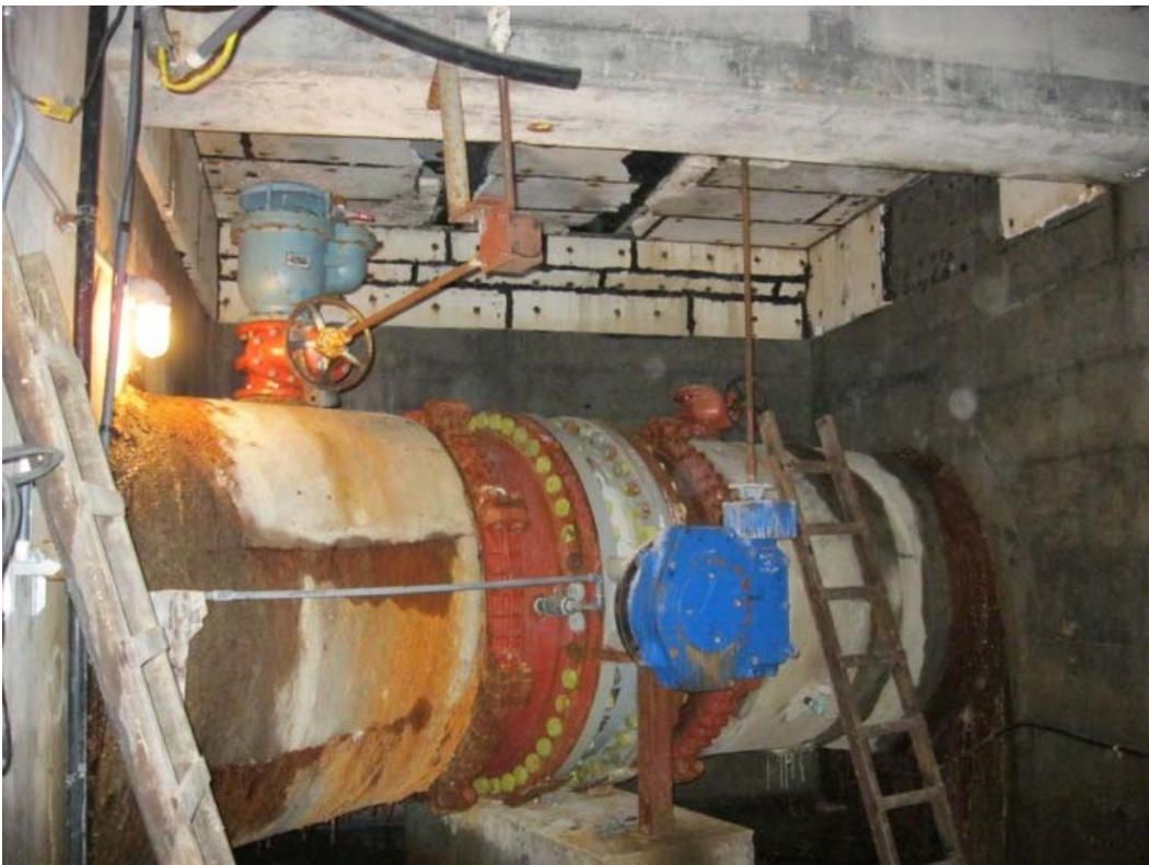
Wilkes Reservoir Valve Pit B – Existing 1350 millimetre Butterfly Valve
