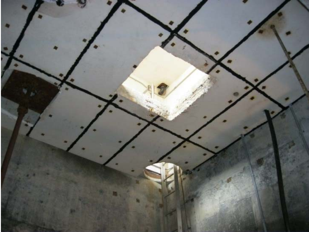
Wilkes Reservoir Valve Pit B – Underside of Operator Floor
