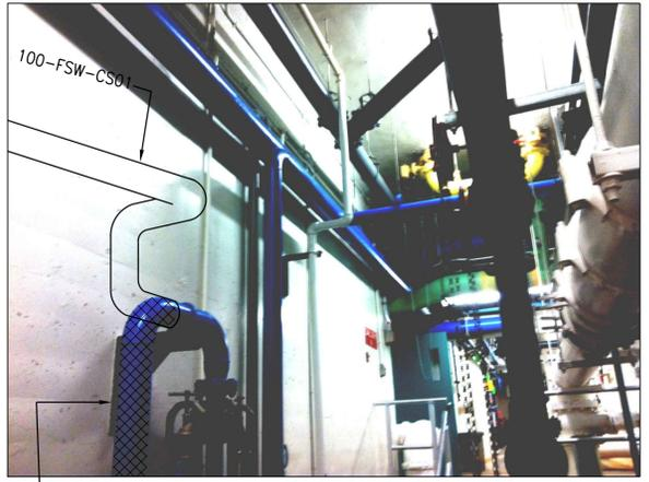
REMOVE 100-FSW-CS01 AS INDICATED CLEAN AND PREP SURFACE WELD AND REROUTE AS SHOWN
