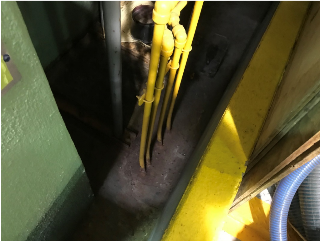
Photo 15 – Diesel Fuel Tanks
