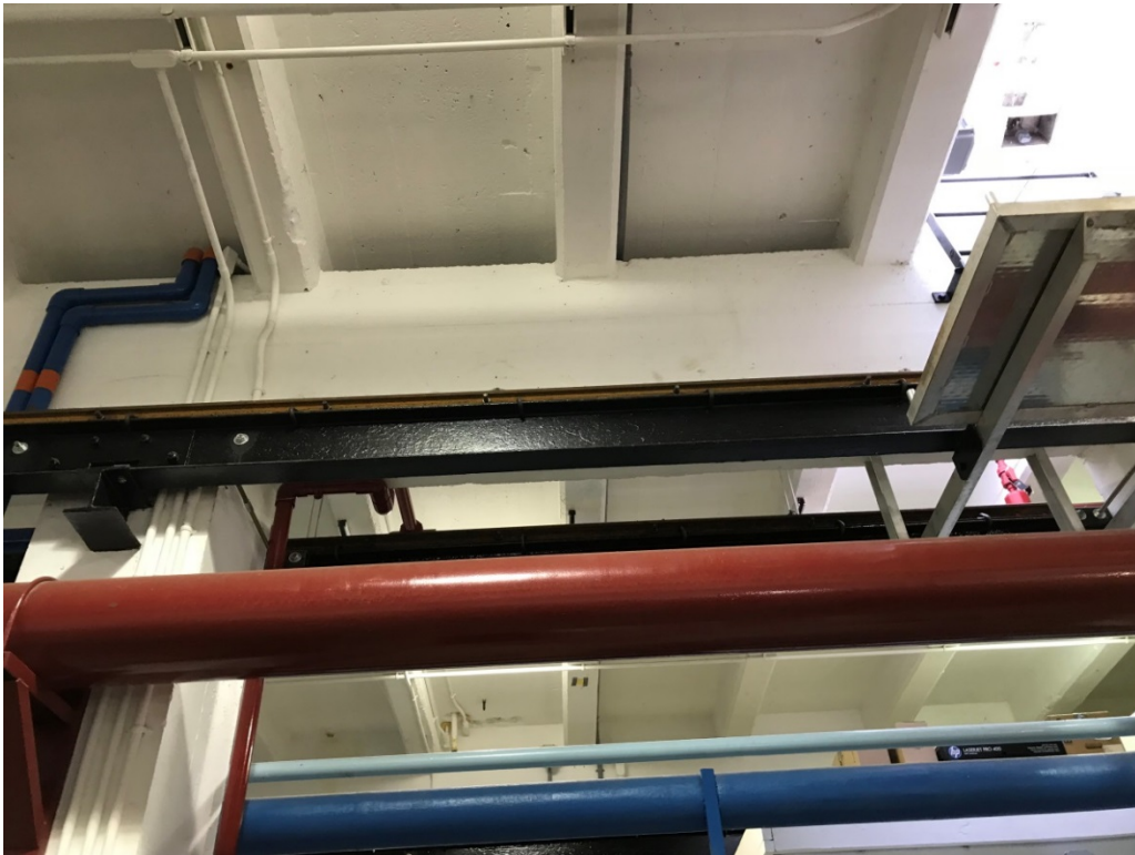
Photo 22 – Gatehouse Skylight and Ceiling
