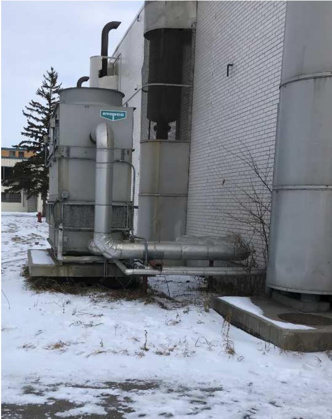
PHOTOGRAPH 1: McPhillips Regional Pumping Station – Main Pumphouse - facing north at the exterior of the building showing the cooling tower fans.
