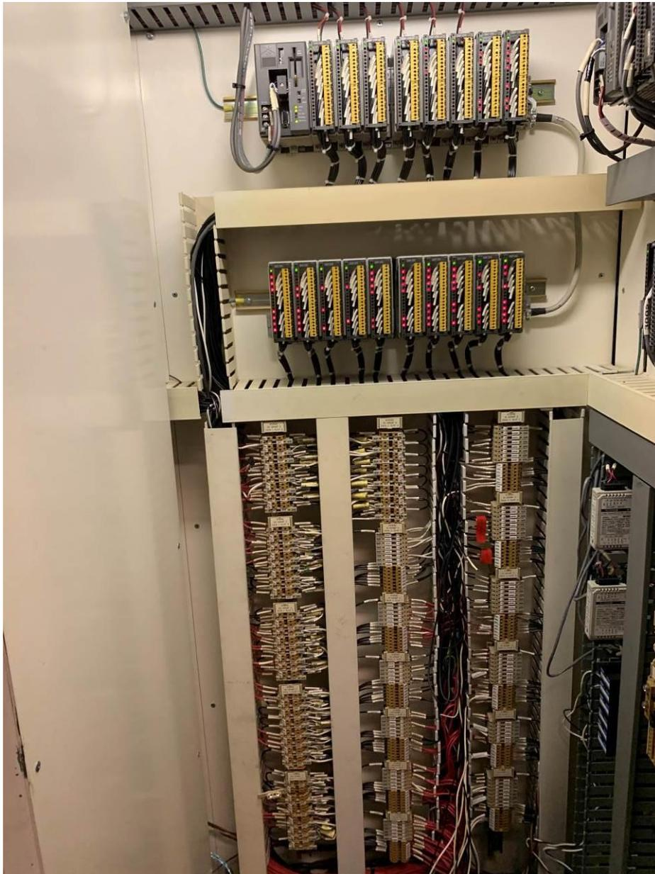
PHOTOGRAPH 18: MacLean RPS main control panel right side interior showing station discrete I/O and terminal block wiring.
