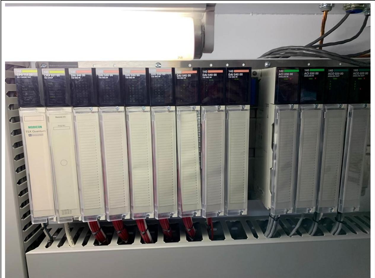
PHOTOGRAPH 34: DBPS UV Master PLC panel remote I/O.
