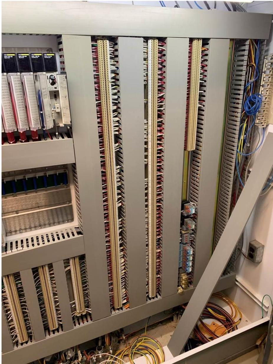
PHOTOGRAPH 39: DCFF main control panel right side interior showing terminal block wiring.
