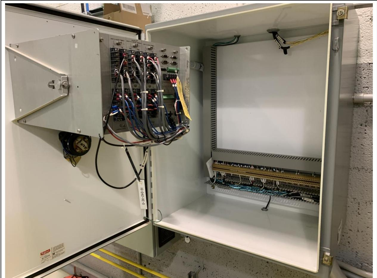
PHOTOGRAPH 71: SLAIF pump room low lift pump #2 control panel PL-59 interior showing the Bently Nevada pump and motor condition monitoring unit wiring.
