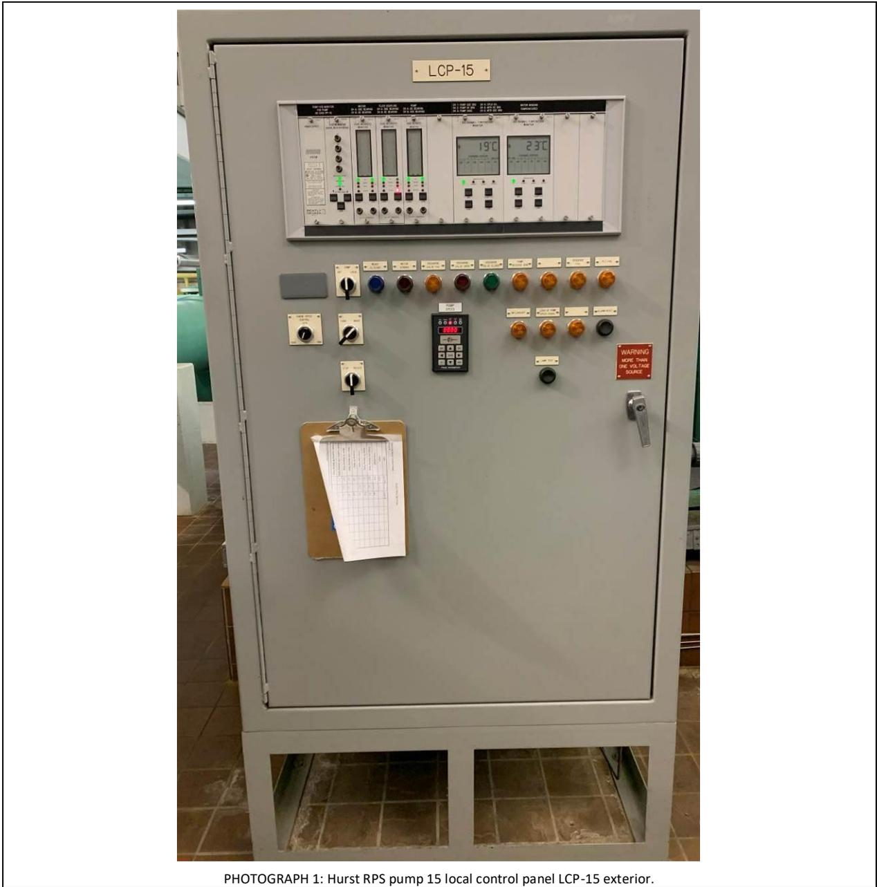
PHOTOGRAPH 1: Hurst RPS pump 15 local control panel LCP-15 exterior.
