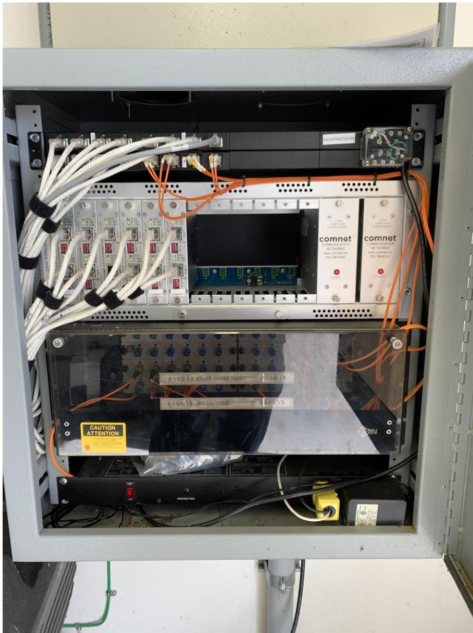
PHOTOGRAPH 86: SLAIF Electrical Shed network panel NP-H800 interior showing the existing network media converter.
