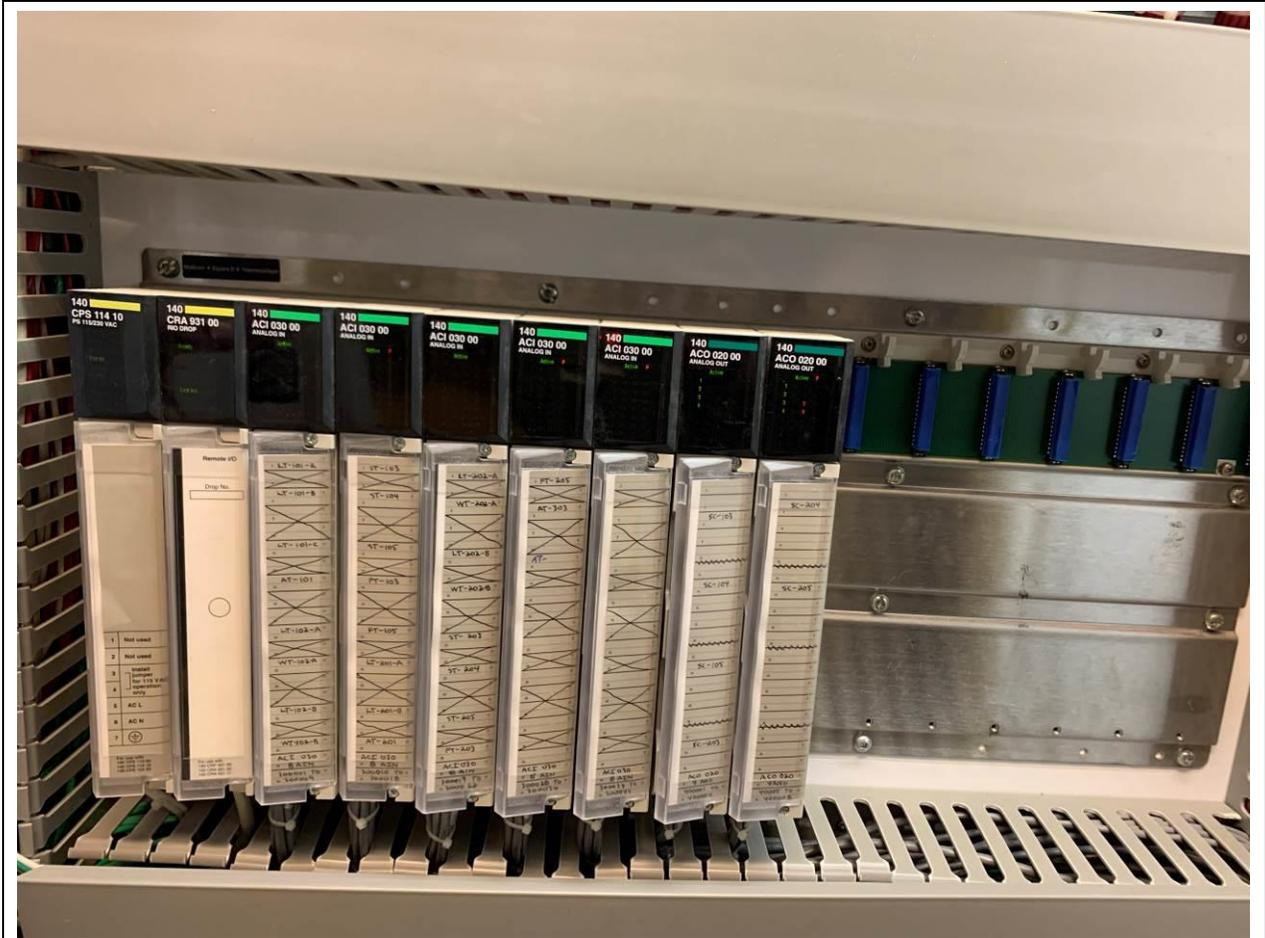
PHOTOGRAPH 41: DCFE main control panel remote I/O.
