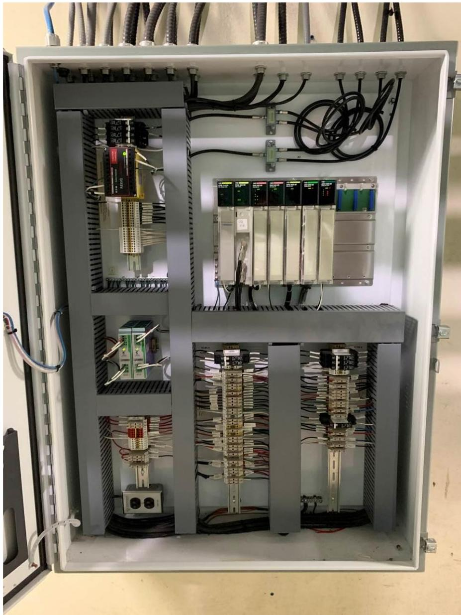
PHOTOGRAPH 22: DBPS local control panel LCP-D12 interior.
