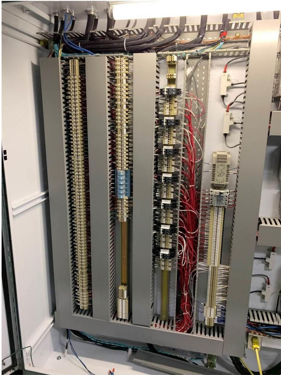
PHOTOGRAPH 32: DBPS UV Master PLC panel left side interior showing terminal block wiring.
