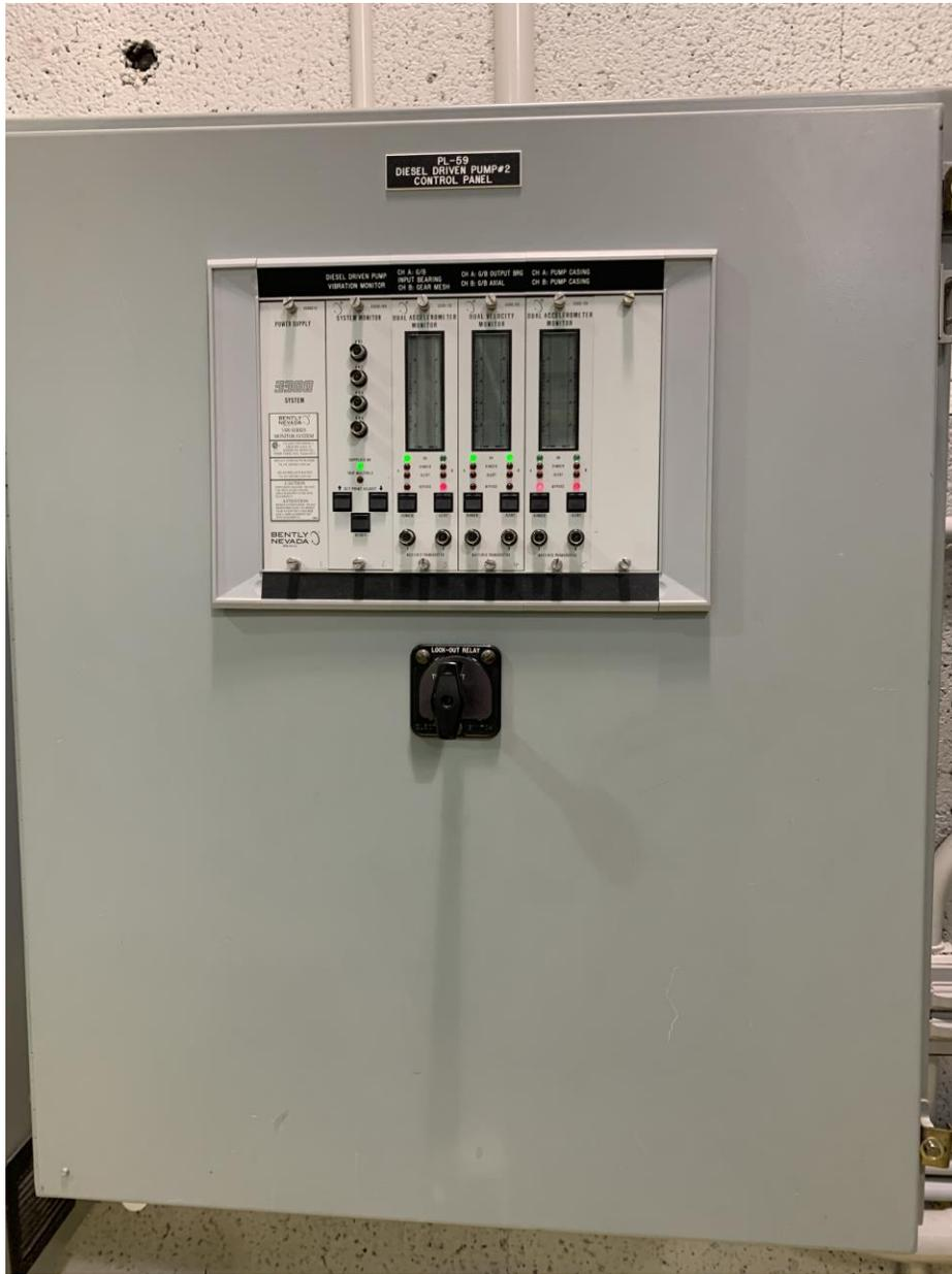
PHOTOGRAPH 69: SLAIF pump room low lift pump #2 control panel PL-59 exterior.
