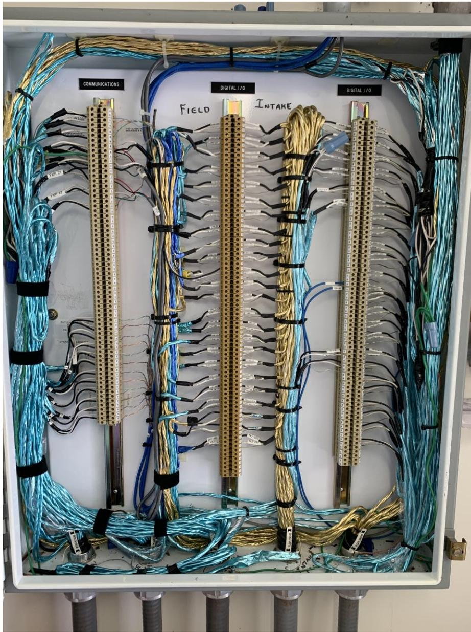
PHOTOGRAPH 88: SLAIF Electrical Shed panel PL-64 interior showing existing terminal block wiring.
