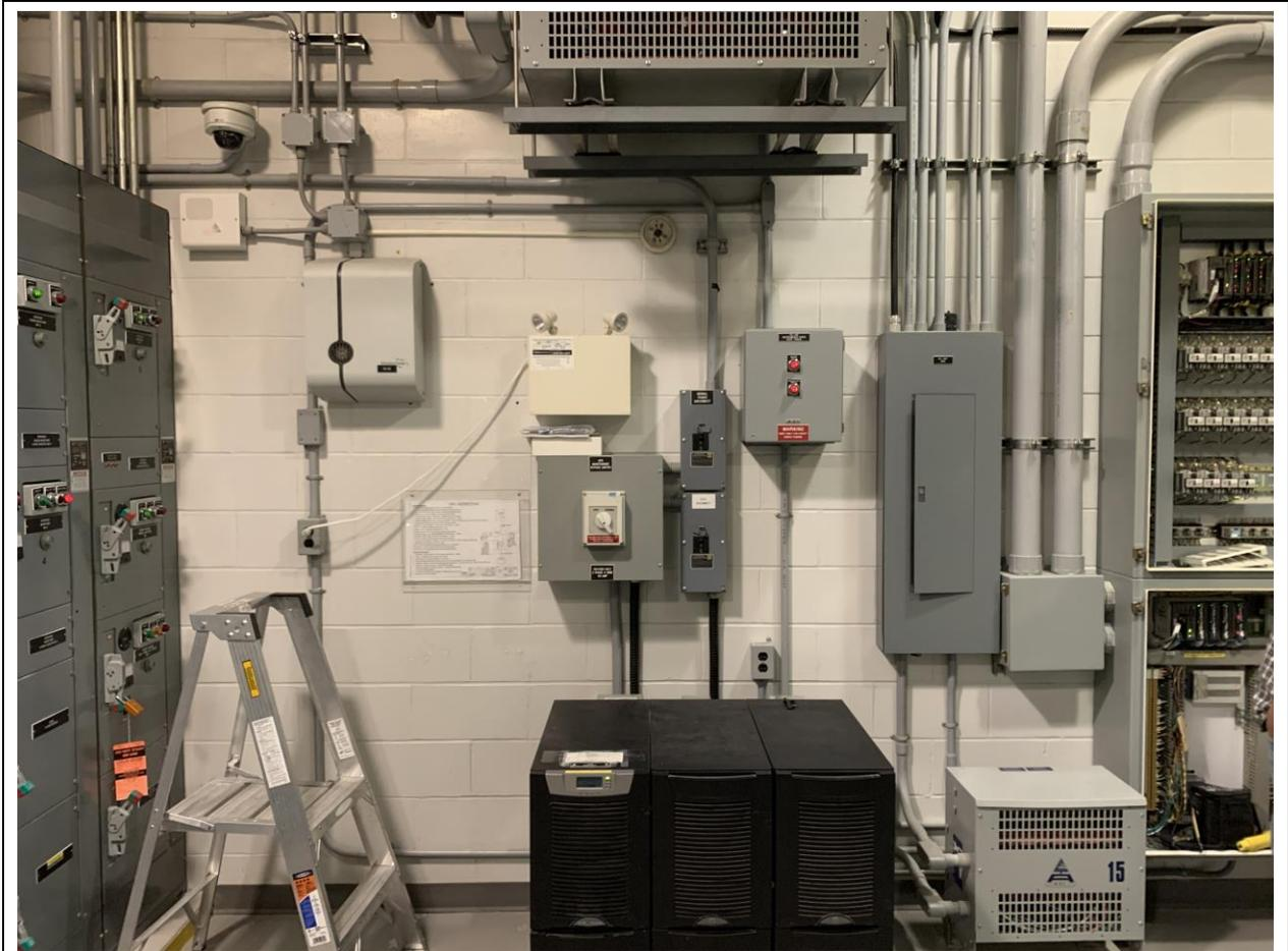
PHOTOGRAPH 58: SLAIF electrical room facing North with MCC on the left and panels ATS PL-43 and PL-43 on the right.
