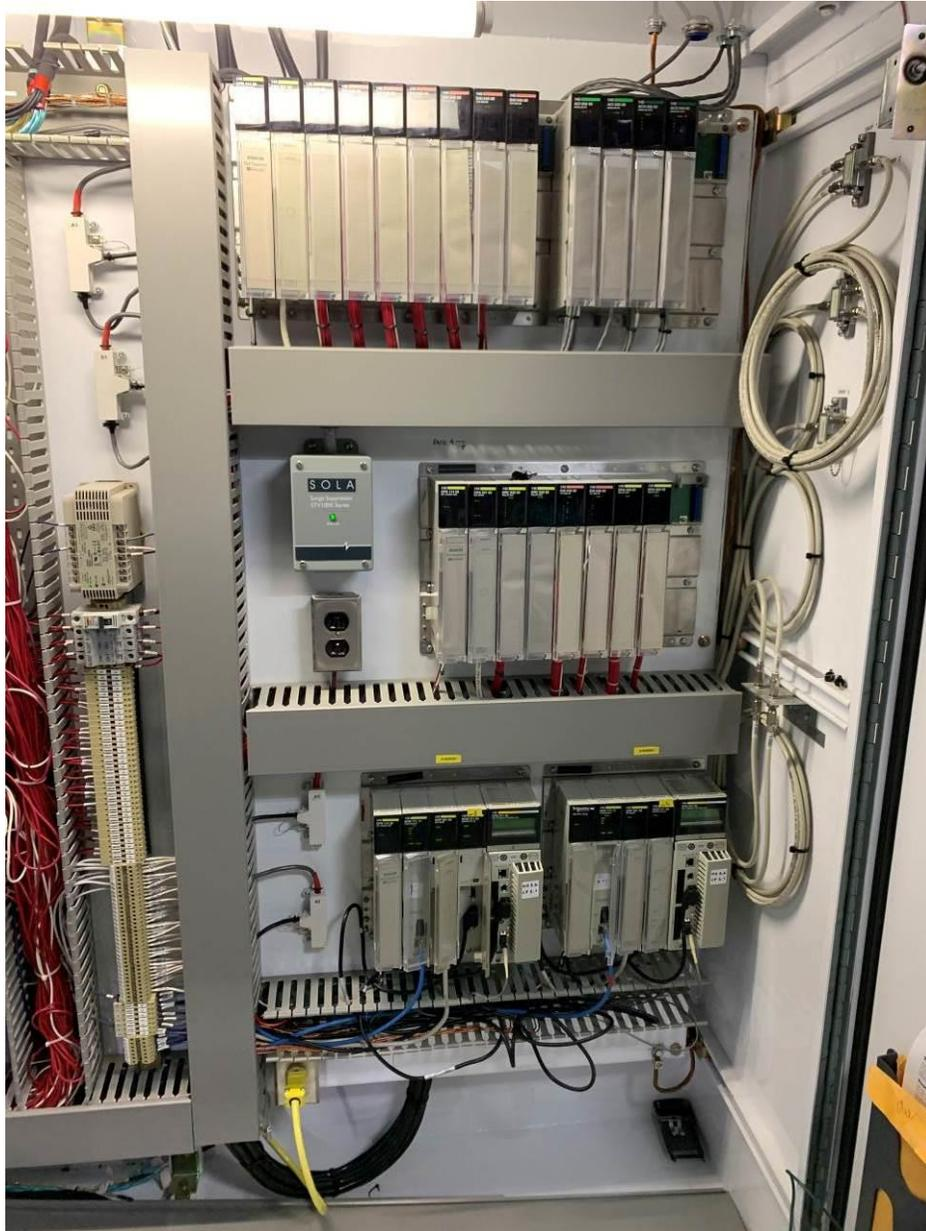
PHOTOGRAPH 33: DBPS UV Master PLC panel right side interior showing redundant PLCs and remote I/O.
