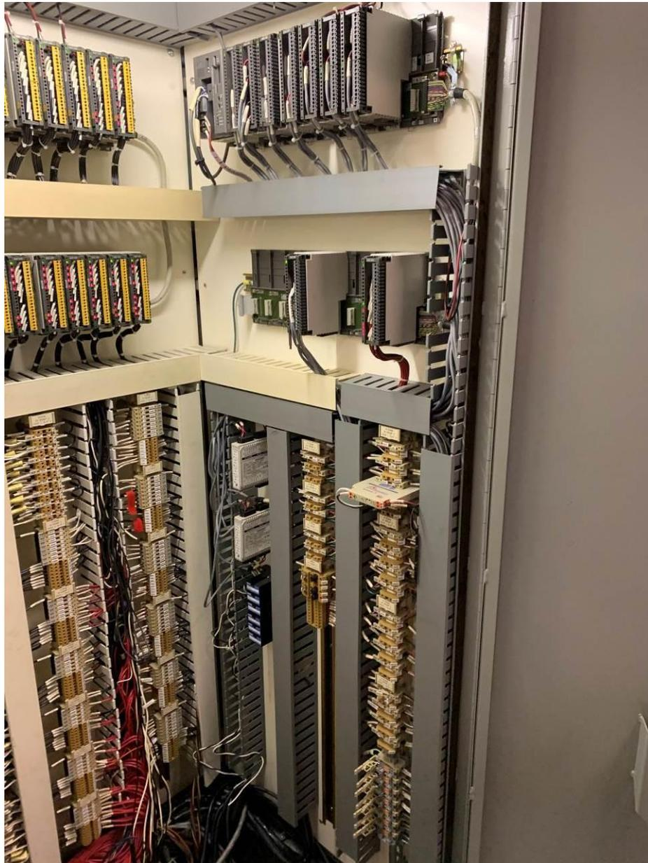
PHOTOGRAPH 19: MacLean RPS main control panel right side interior showing station analog I/O and terminal block wiring.
