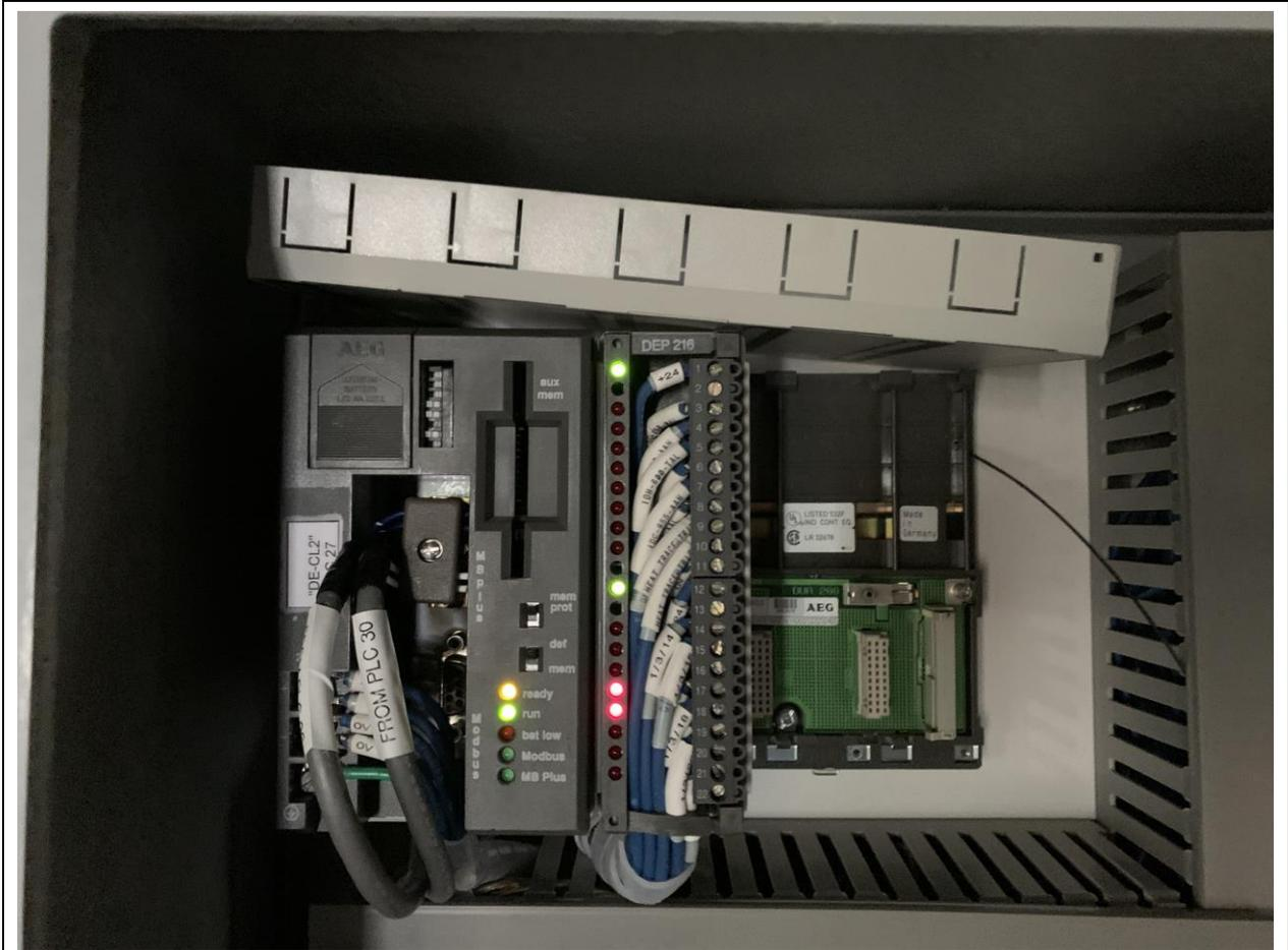
PHOTOGRAPH 80: SLAIF Dechlorination Building alarm panel PL-42 PLC 27.
