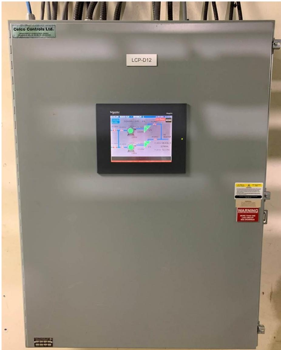
PHOTOGRAPH 21: DBPS local control panel LCP-D12 exterior.
