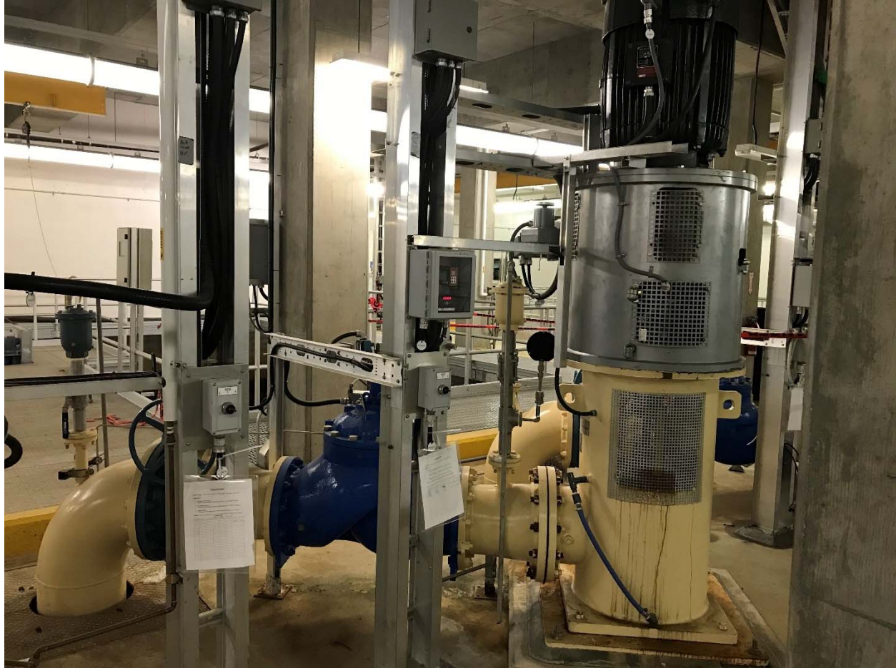
Photograph 1: Deacon Water Treatment Plant MagDrive Supernate Pump
