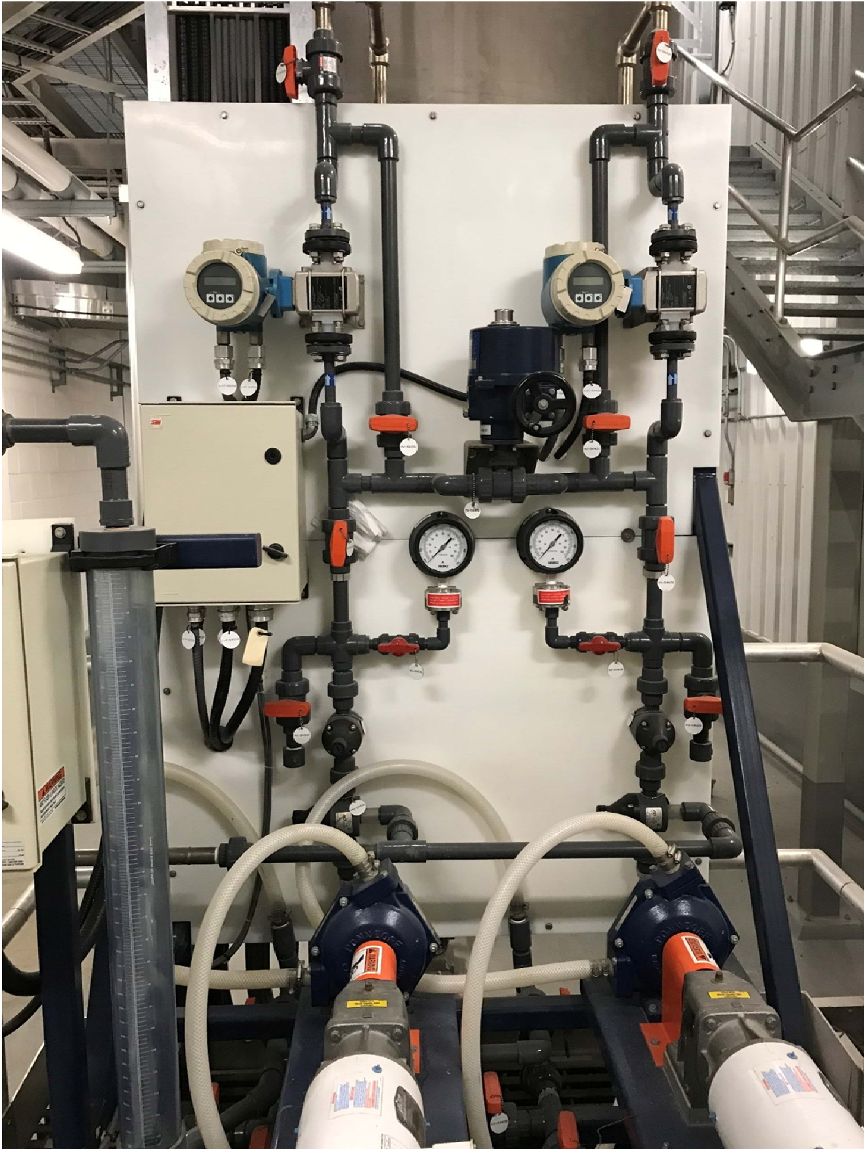
Photograph 6: Deacon Water Treatment Plant Existing Ammonia Dosing Skid
