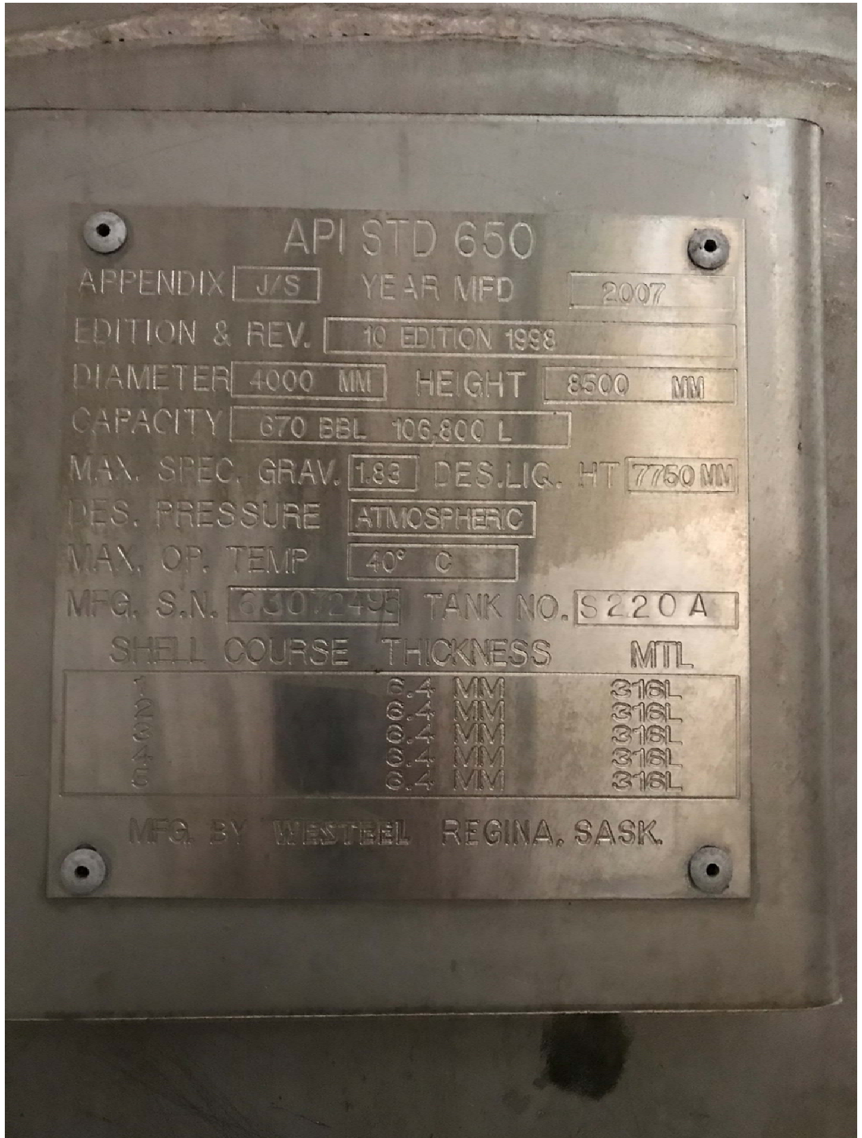
Photograph 4: Deacon Water Treatment Plant Existing Sulphuric Acid Tank Nameplate
