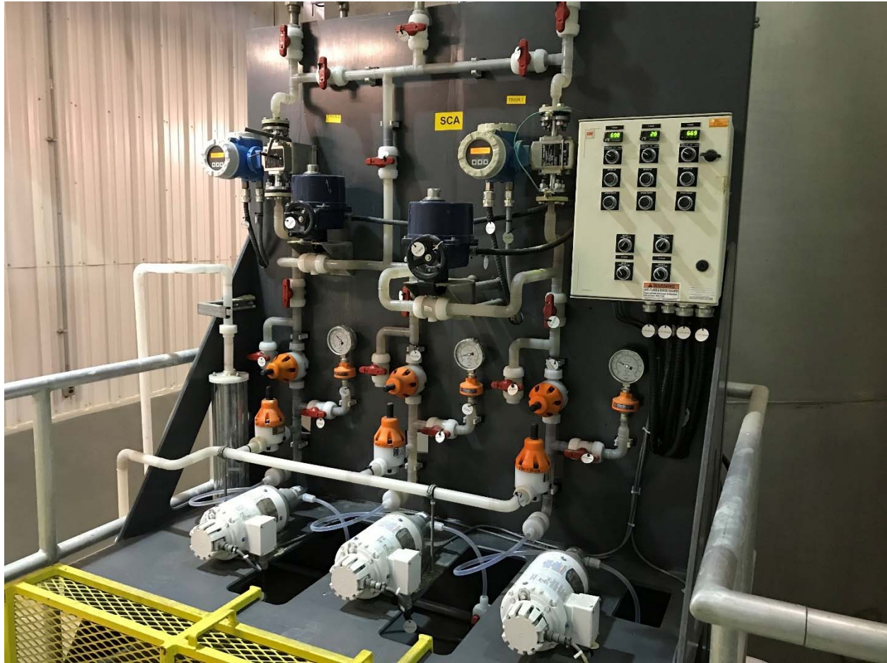
Photograph 3: Deacon Water Treatment Plant Existing Sulphuric Acid Dosing Skid
