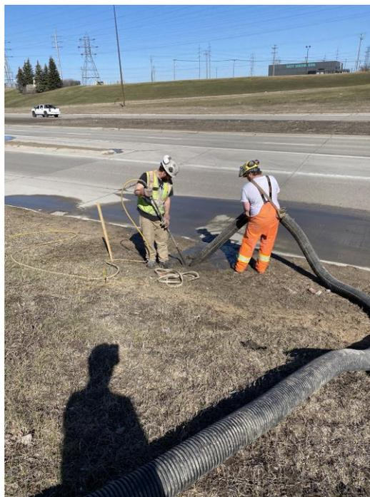
Photo 2. Looking west, hydro-excavation at the toe
