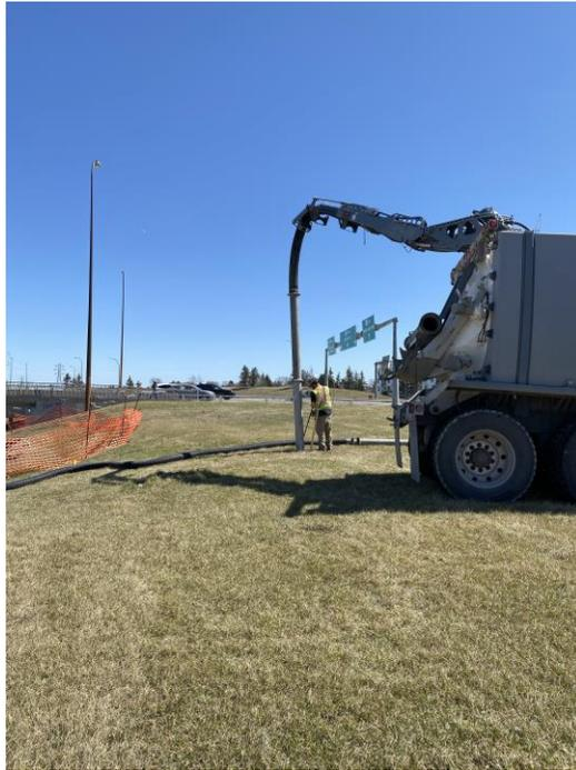
Photo 5. Looking east, hydro-excavation at the cress
