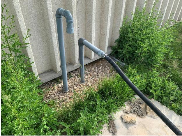
Figure 3: Existing corrugated well to be replaced. PVC piping to remain in place.
