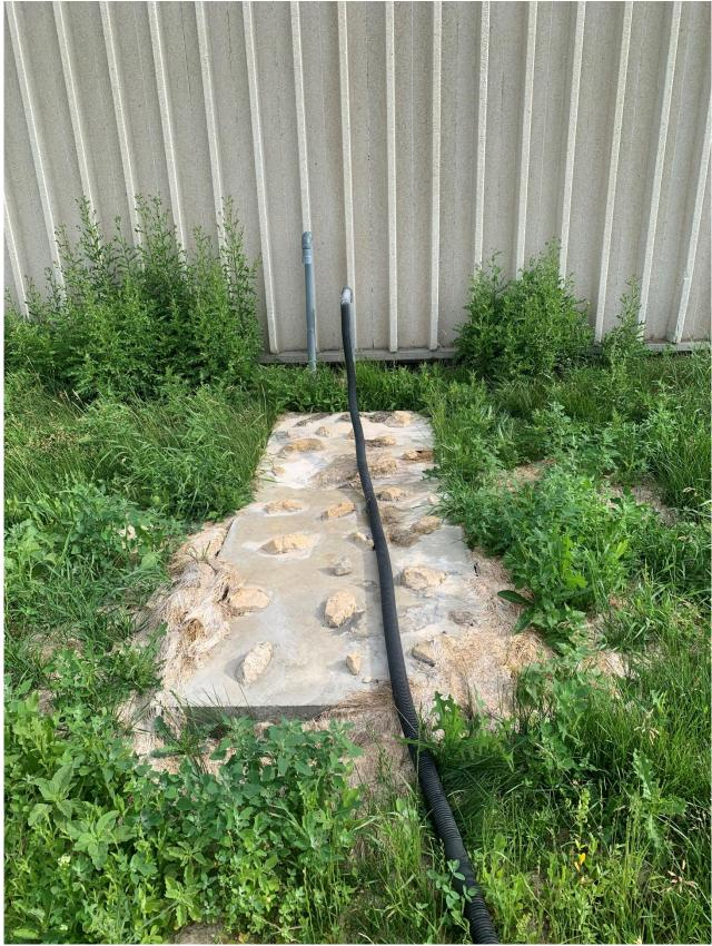
Figure 1: Existing sump discharge swale to be removed.
