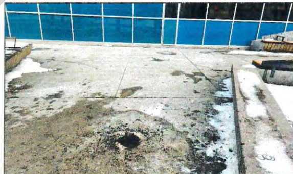
PHOTOGRAPH 2: FACING EAST, SHOWING THE TEST HOLE AFTER COMPLETION OF DRILLING.
