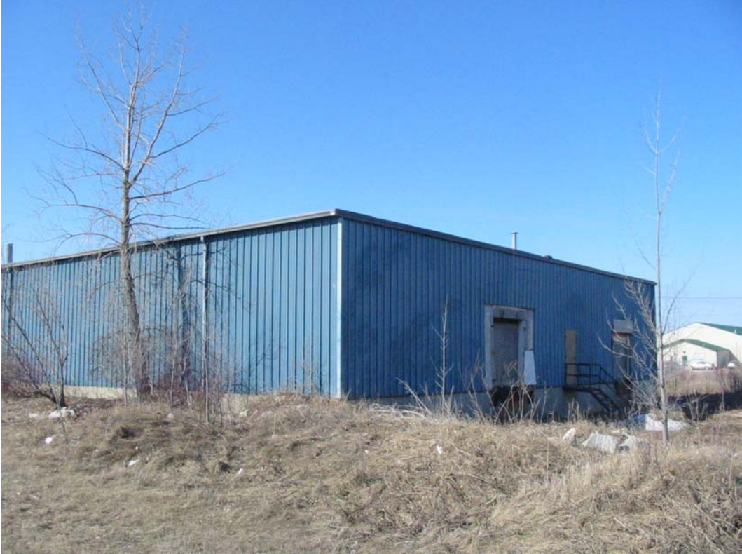
215 Panet Rd –North East
