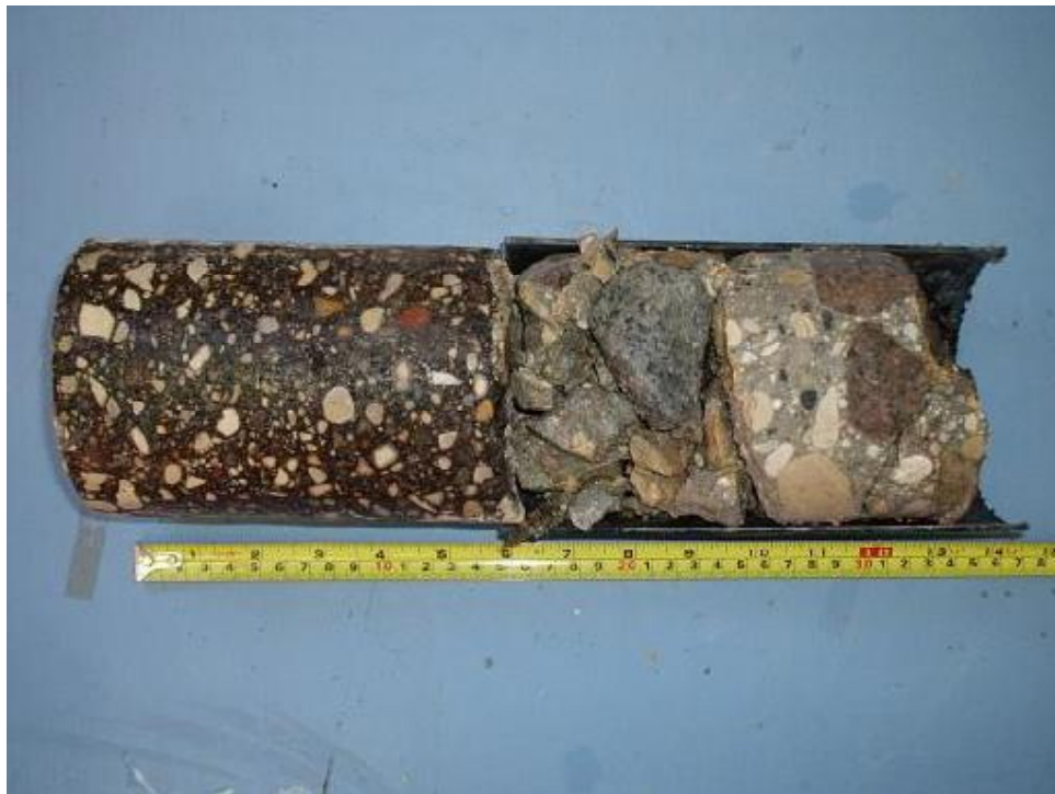
Photo No. 4: Center lane, 17 m north from Jackson Avenue
