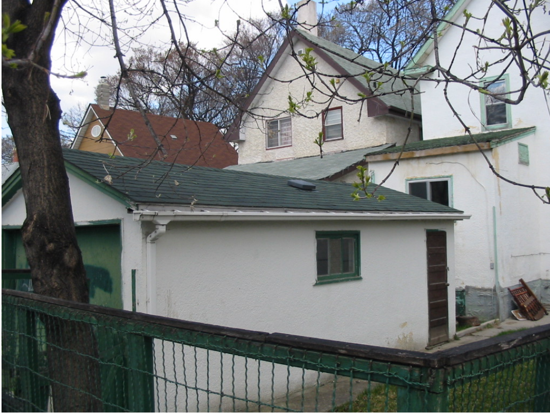
148 Alfred Ave – Garage
