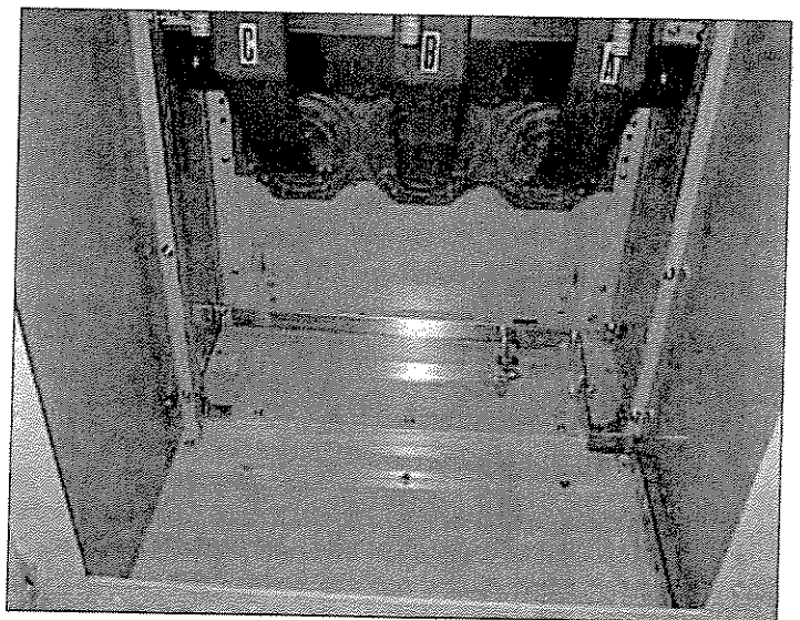
Figure 4. Ground Bus Installation.
