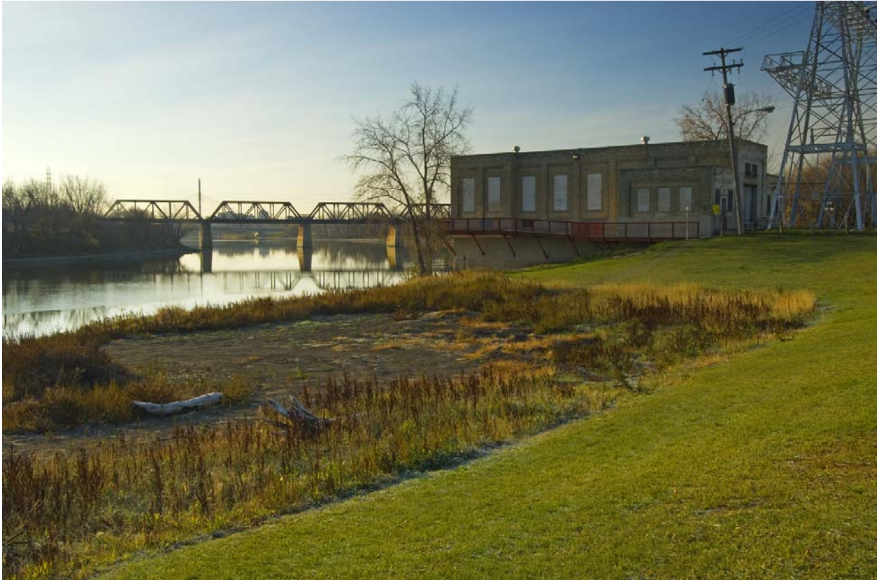
The Northern Façade of Building and view southward
