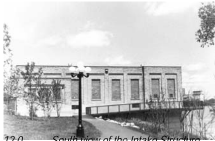
12.0 South view of the Intake Structure
