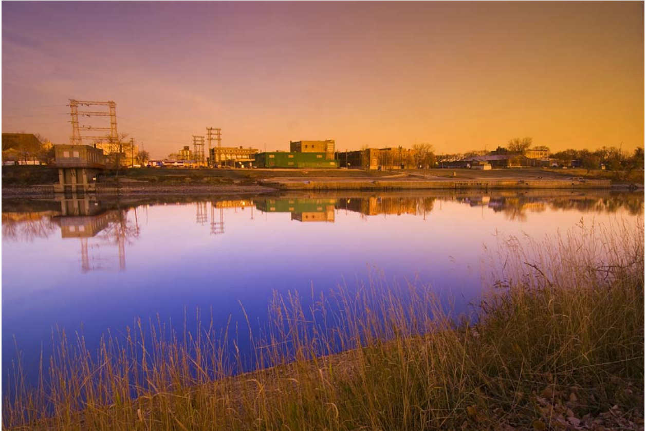
View Westward across the Red River showing the Alexander Dock and Harbourmaster Building
