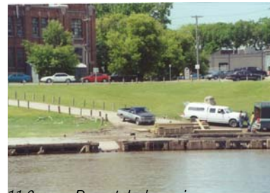
11.0 Recent dock repairs
