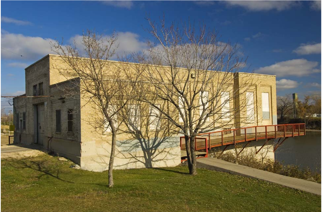
The Southern Façade and view northward
