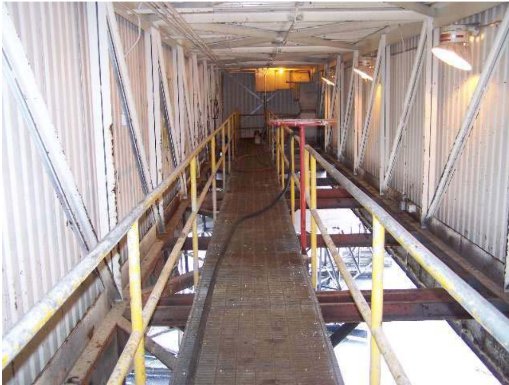
Photo 3-14 Clarifier Walkway & Enclosure
