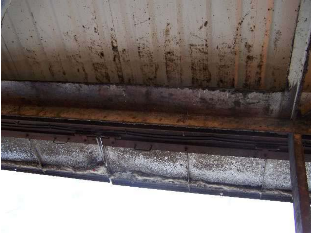
Photo 3-15 Enclosure Hinged Scum Blade Access Panels
