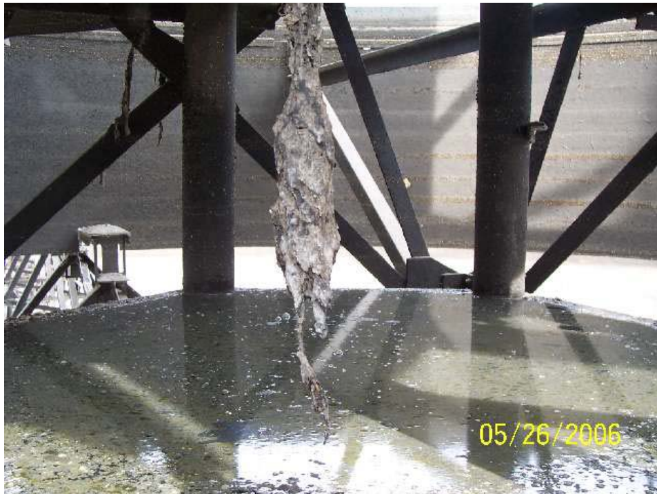
Photo 3-2 Top of Concrete Clarifier Influent Pipe/Base
