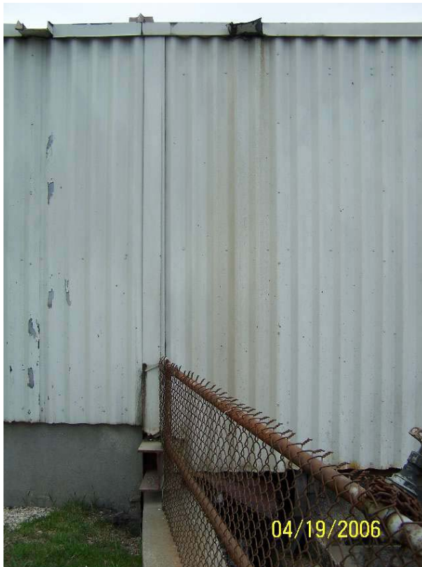
Photo 2-4 Clarifier Walkway Enclosure Connection
