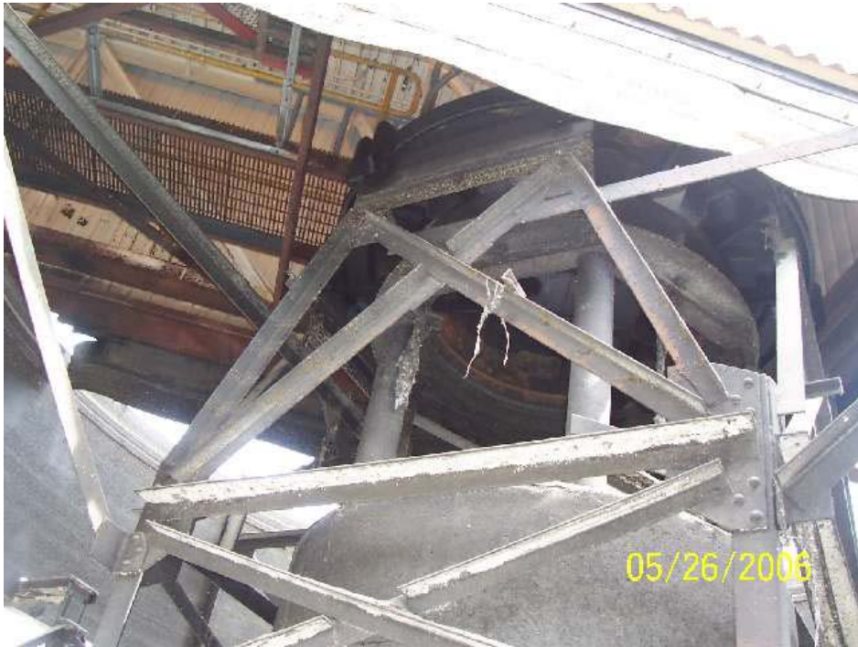
Photo 3-1 Concrete Clarifier Influent Pipe/Base
