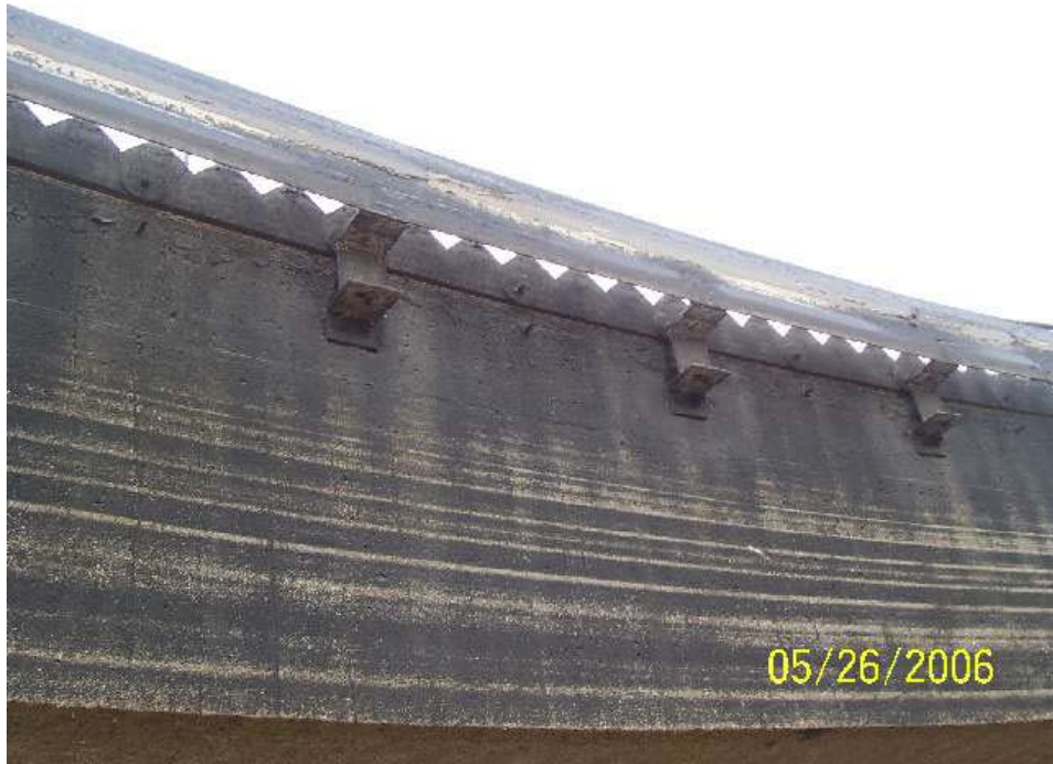
Photo 3-3 Effluent Weir & Scum Baffle
