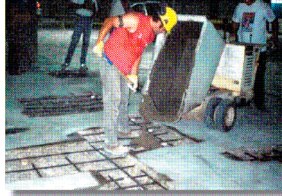
Complete the repair with compatible repair material.
