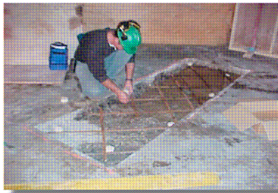
Anodes installed and ready for repair.
