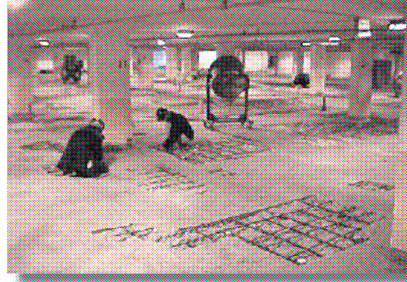
Anodes should be placed around the perimeter of the patch. (See data sheet for spacing guidelines)
