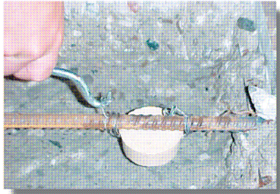
Tie the anode on the side or beneath the rebar providing minimum 3/4 in. cover and clearance on all sides
