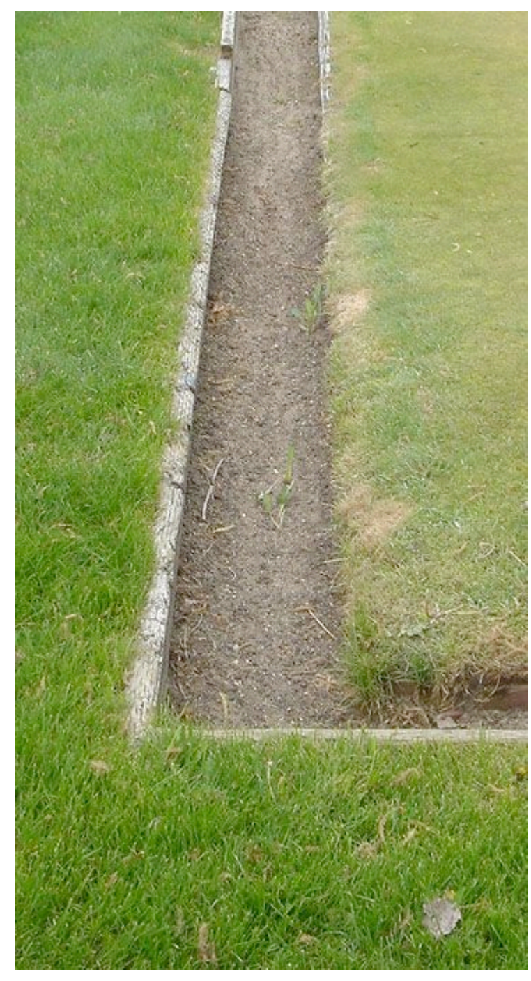
3 Typical Existing Ditch L1
