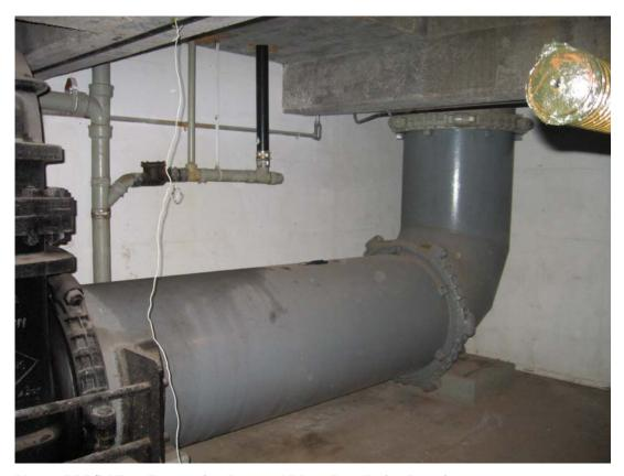
Photo - PRPS 1 East Forcemain - Proposed Meter Installation Location
