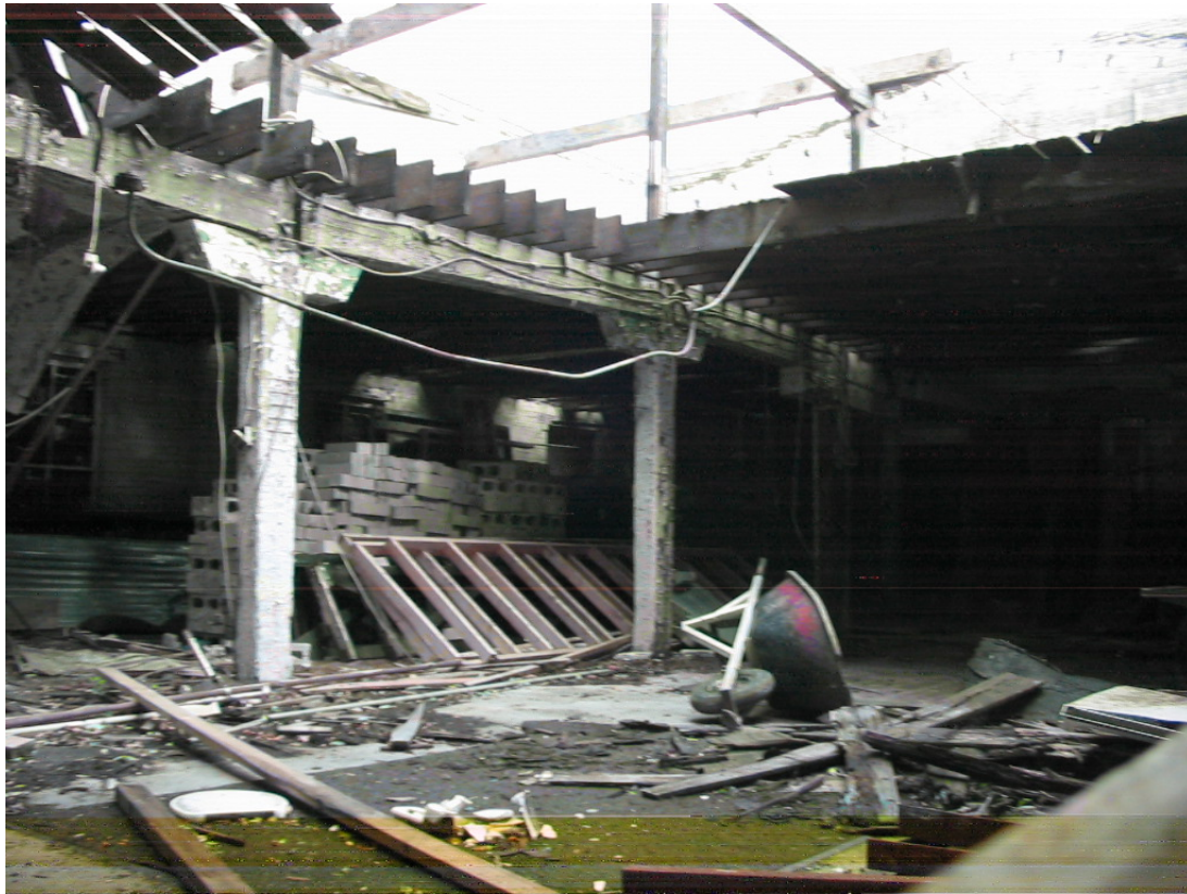
Inside view – no roof
