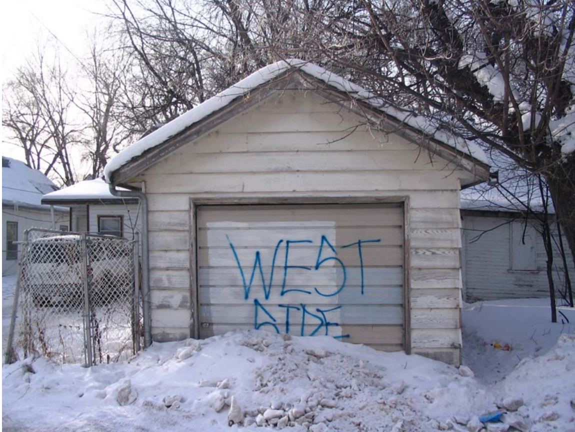
Front of garage from back lane
