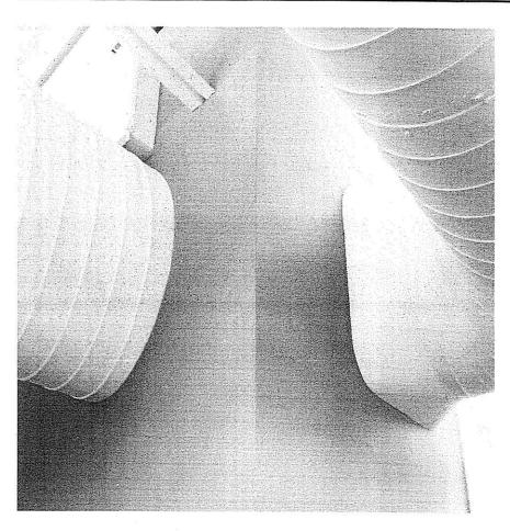
**4.** Provide an elbow silencer within the boiler room on the duct between gridlines P and Q, to reduce the transmission of ductborne noise between the boiler room and the library. Refer to photographs below.
