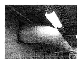
**5.** Revise the duct supply plenum from AHU-4, increase the thickness of the duct to minimum 18 gauge. The revised plenum is to be acoustically lined. The plenum is to be enlarged to increase the volume. Relocate the existing light fixture to suit the installation of the revised supply plenum. Provide silencers at each duct take-off. Refer to photographs below.
