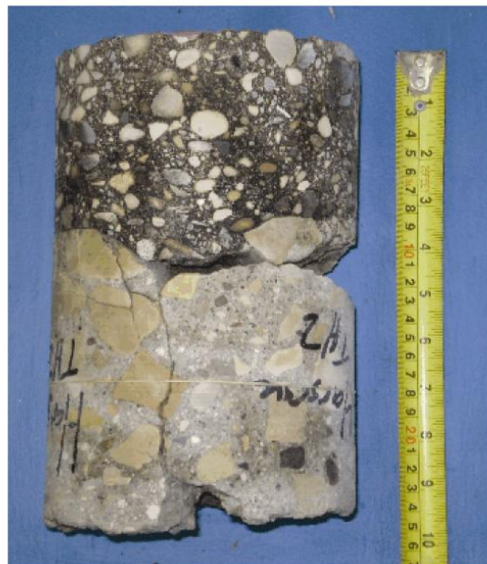
Core sample from Testhole TH2
