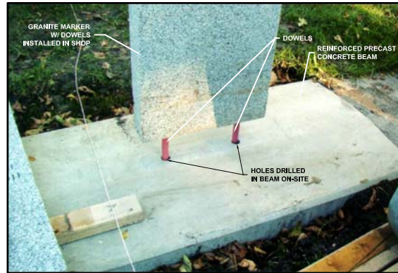
PHOTO OF TYPICAL MARKER MOUNTING
