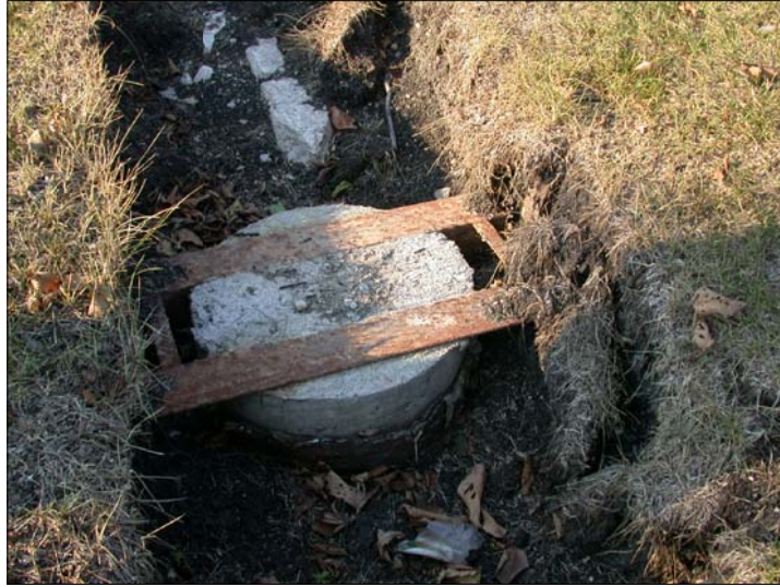
PHOTO OF EXISTING STEEL SUPPORT & CONCRETE PIER
