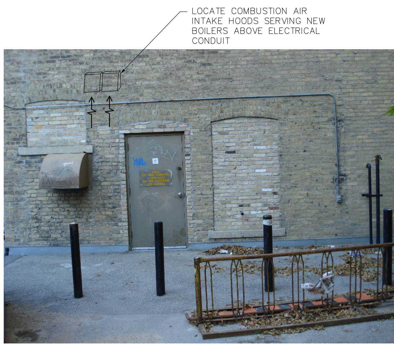
1 COMBUSTION AIR INTAKE M03 NTS
