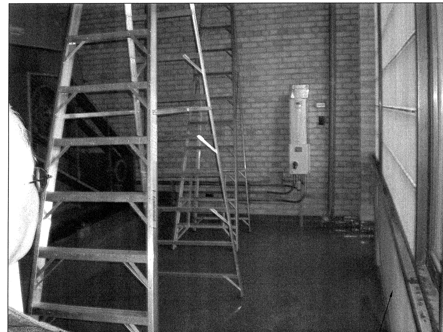
2 PHOTO #1 SCALE: NTS THIS WALL CONTAINS ASBESTOS. DO NOT FASTEN OR SUPPORT PIPING, EQUIPMENT, ETC. TO WALL ON GRID LINE '3'. SEE NOTE 5.
