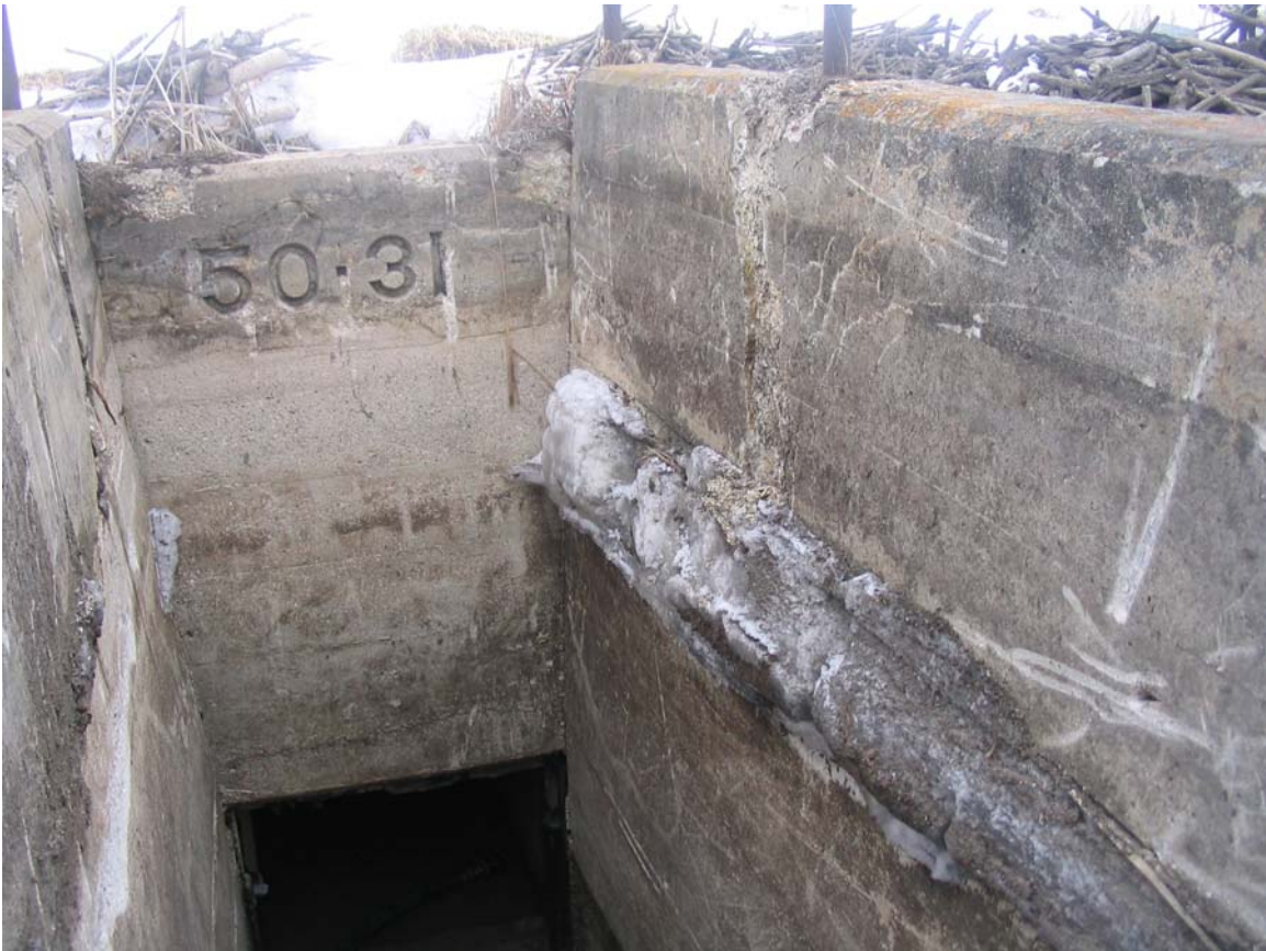
Mile 50.31 South Headwall
