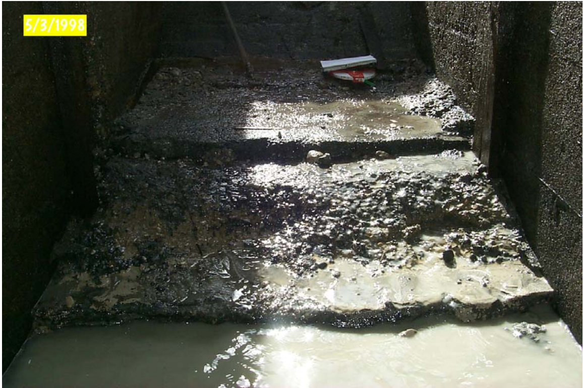
Mile 50.31 Lower Box Benching
