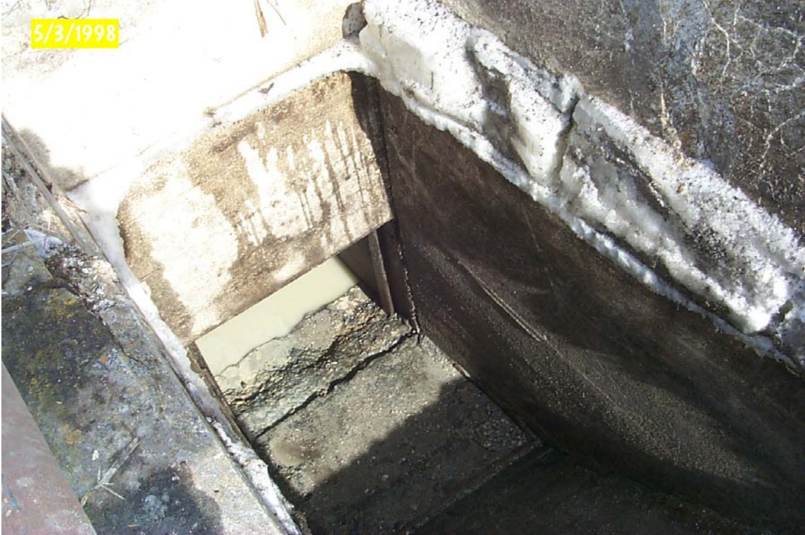
Mile 50.31 North Side Lower Box
