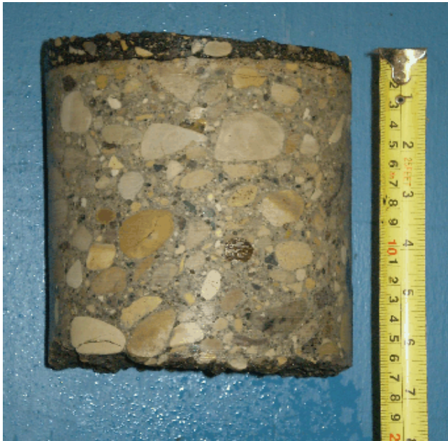
Pavement core from Testhole TH 1
