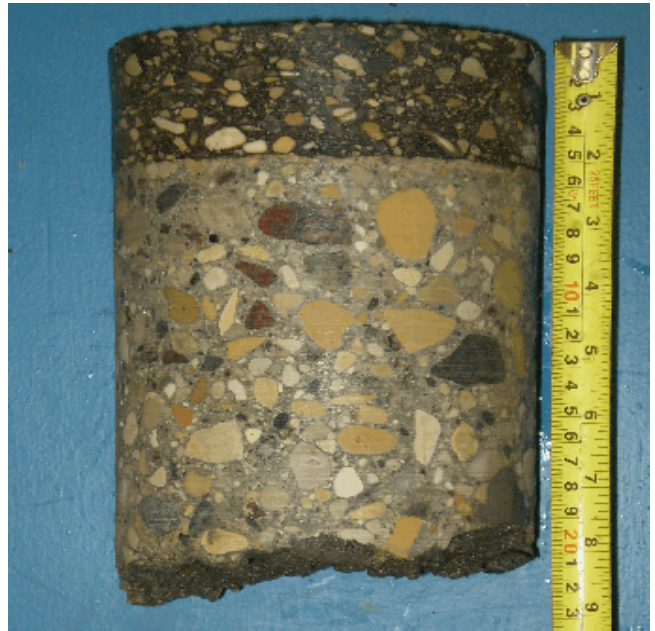
Pavement core from Testhole TH 10
