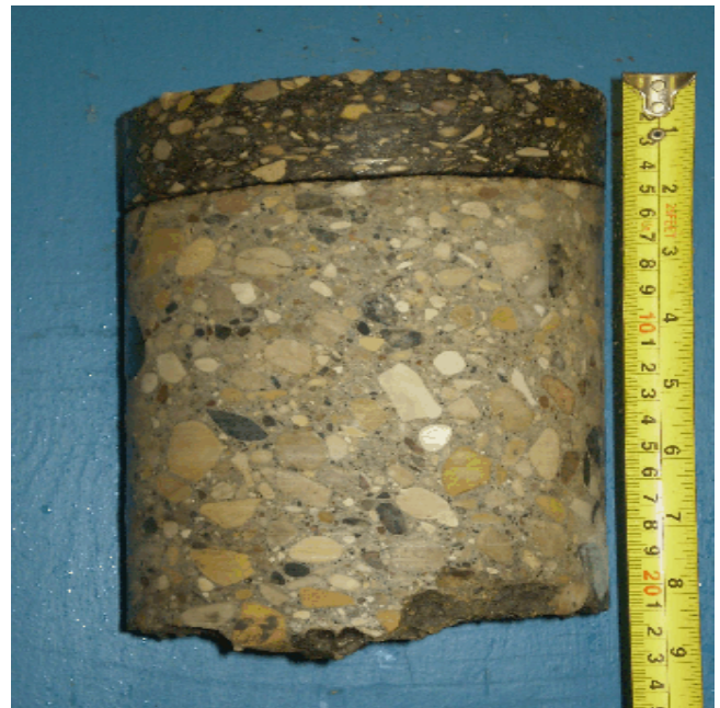
Pavement core from Testhole TH 4
