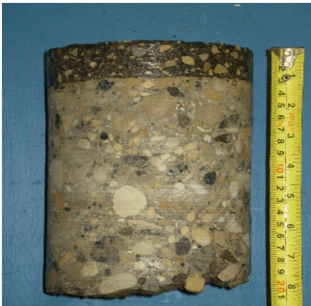
Pavement core from Testhole TH 7
