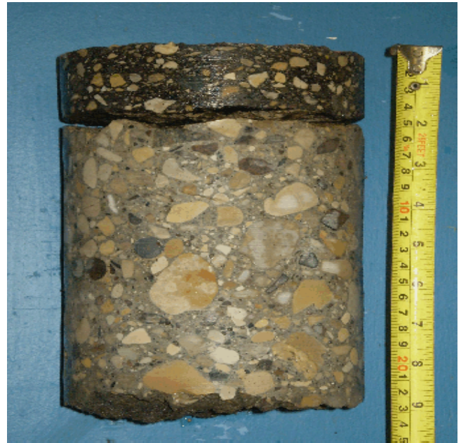
Pavement core from Testhole TH 6
