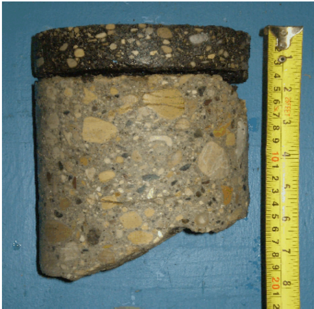
Pavement core from Testhole TH 5
