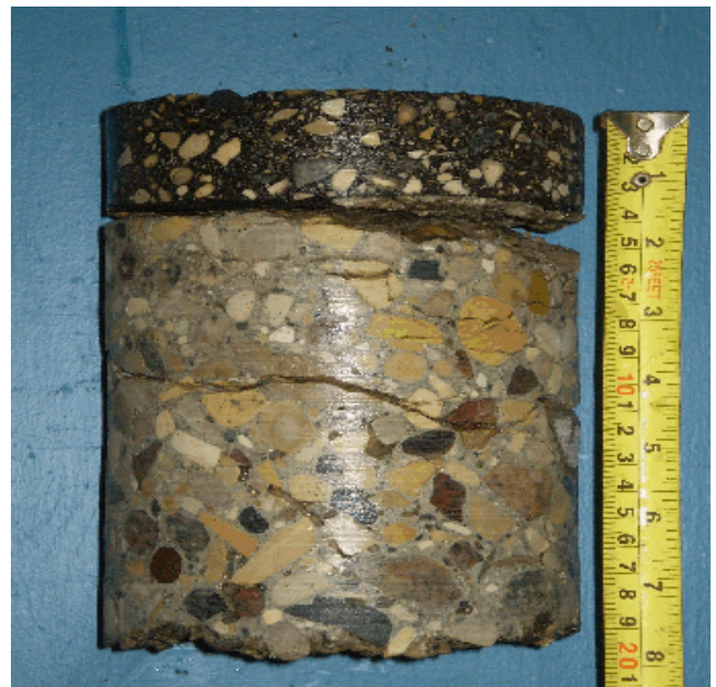
Pavement core from Testhole TH 8
