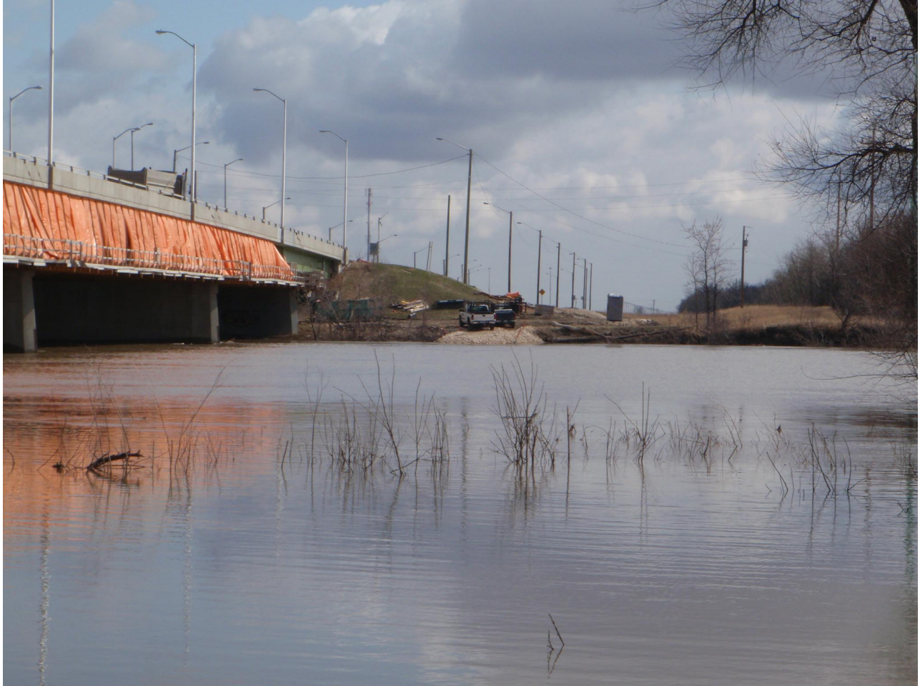
South Perimeter Bridge (East Side): Site access from Perimeter Highway. Looking east from west side of bridge.
