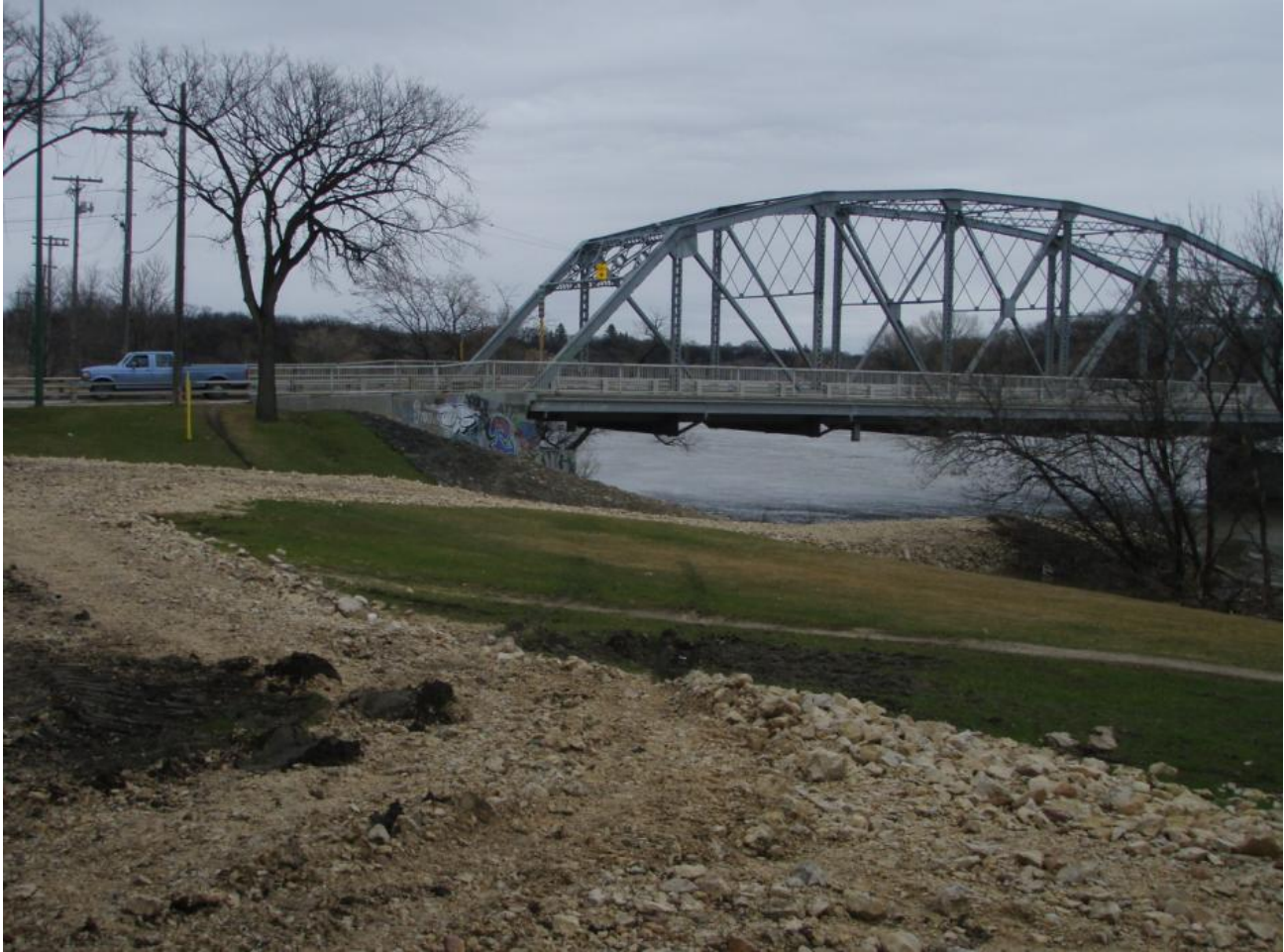
Redwood Bridge: Limestone at west abutment, south of bridge.
