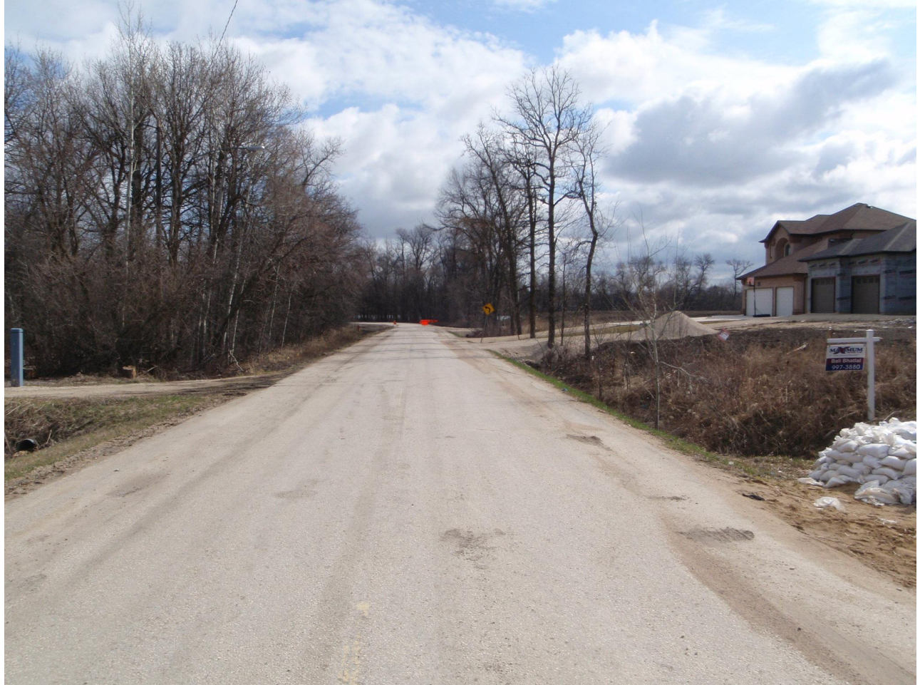
South Perimeter Bridge (West Side): Site access from Cloutier Drive, south of bridge.
