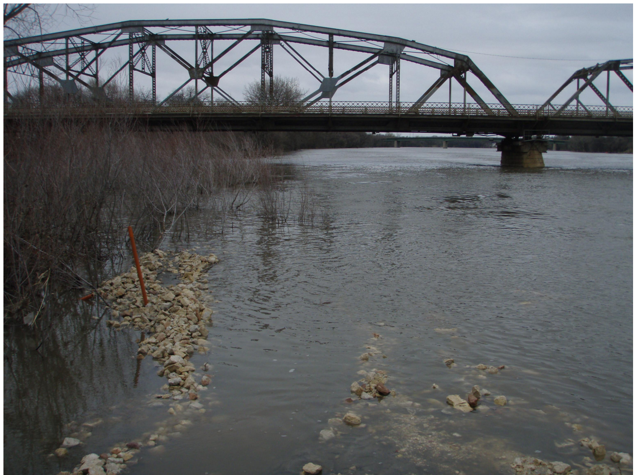
Louise Bridge: Limestone at south abutment, east of bridge.
