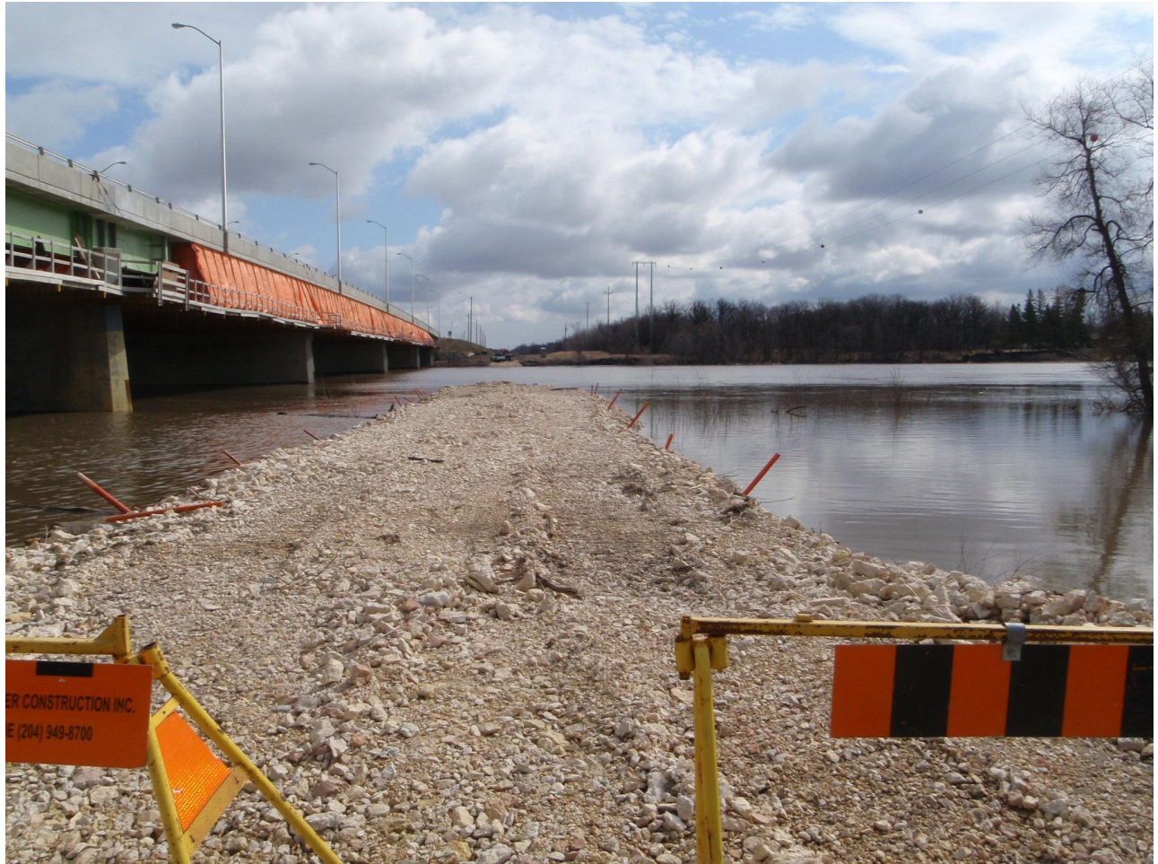
South Perimeter Bridge (West Side): Limestone south of bridge.
