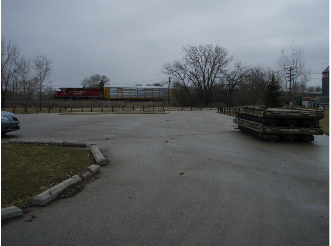
Louise Bridge: Site access from Higgins Avenue.
