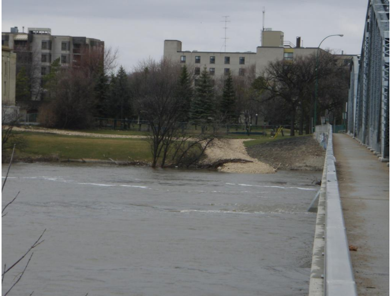
Redwood Bridge: Limestone at west abutment, south of bridge. Looking west from east side of bridge.
