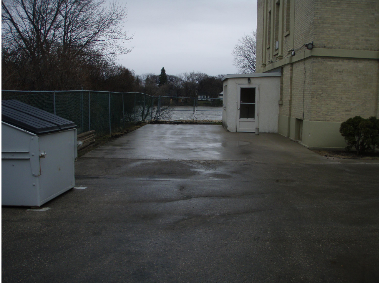
Redwood Bridge: Site access from Sisters Servants of Mary Immaculate parking lot on Aberdeen Avenue.
