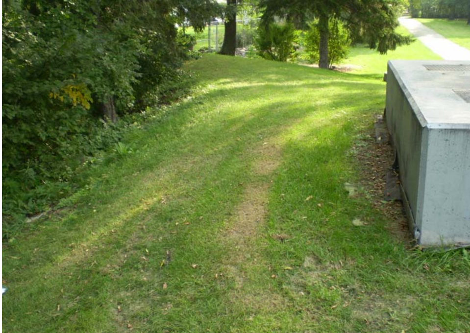
Photo 23- Elmwood Park: Ruts from vehicles by gate chamber.
