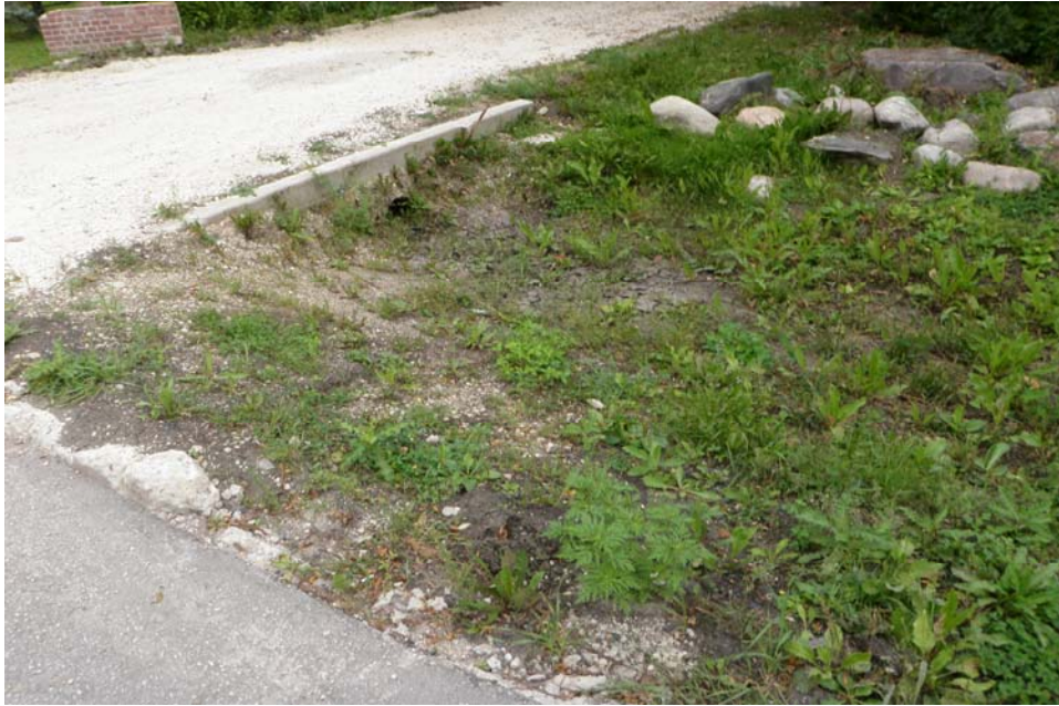
Photo 9 – Bonner at Bunns Creek: Ditch from #275 – 277, one of culverts to be cleaned and curb repairs
