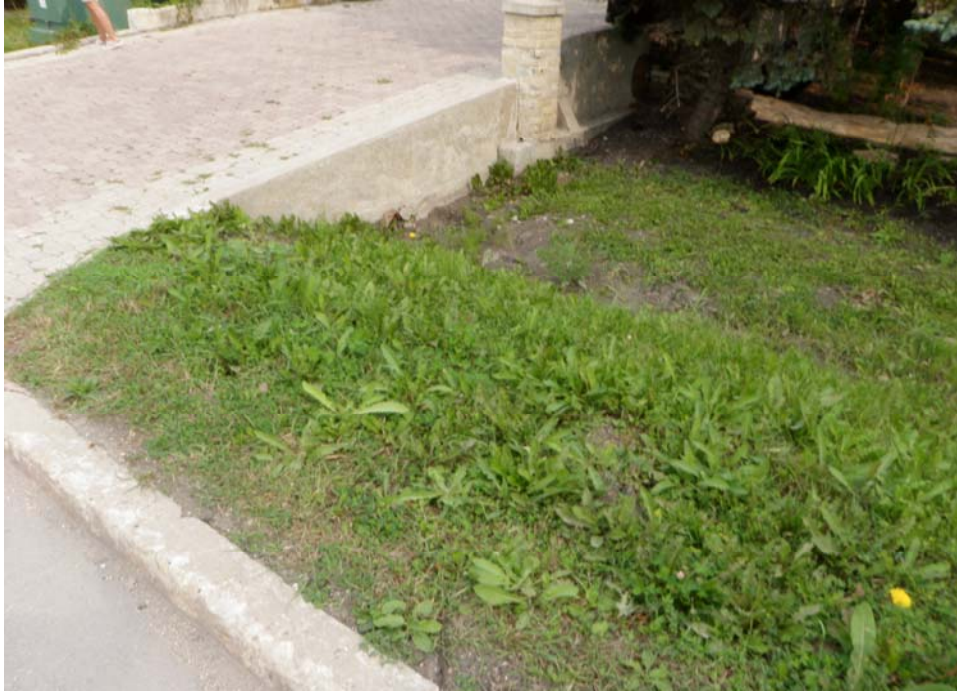
Photo 13 – Bonner at Bunns Creek: Ditch between #273 – 275, culvert to be cleaned
