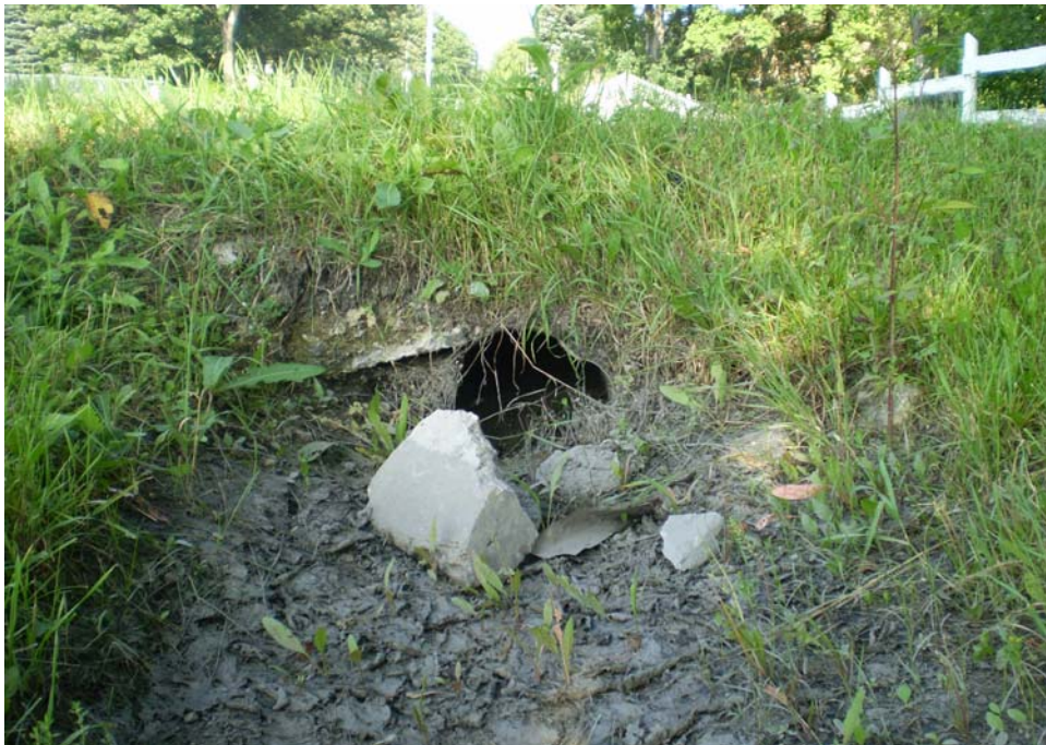
Photo 16 -Bonner at Bunns Creek: Culvert to be cleaned beneath driveway of #271
