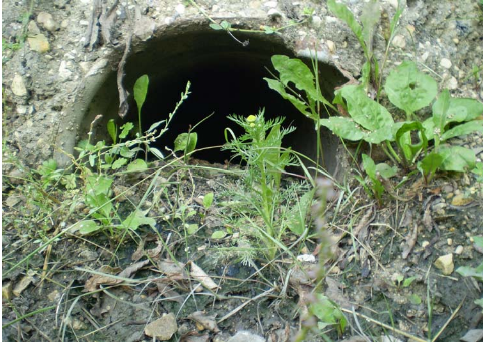
Photo 17 – Bonner at Bunns Creek: Culvert to be cleaned beneath driveway of #277
