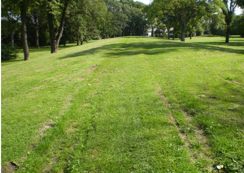
Photo 21 -Elmwood Park: Rutted area top of berm.
