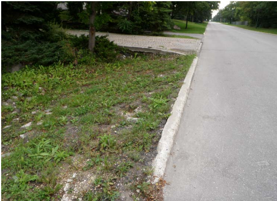
Photo 10- Bonner at Bunns Creek: Ditch from #275 – 277
