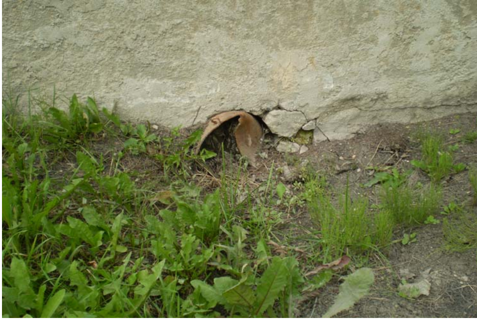
Photo 19 - Bonner at Bunns Creek: Culvert to be cleaned beneath driveway of #273
