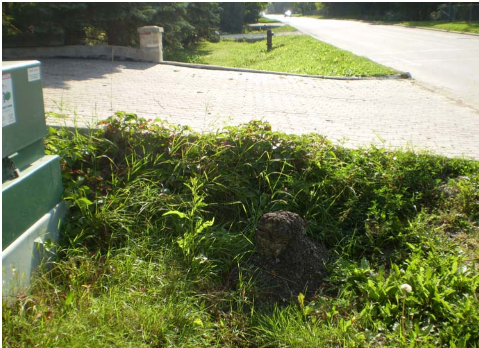
Photo 18 – Bonner at Bunns Creek: Culvert to be cleaned beneath driveway of #273
