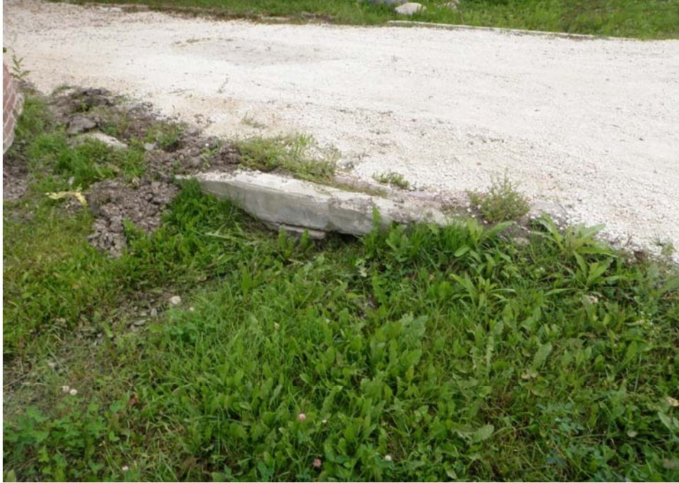
Photo 15 – Bonner at Bunns Creek: Culvert to be cleaned beneath driveway of #275
