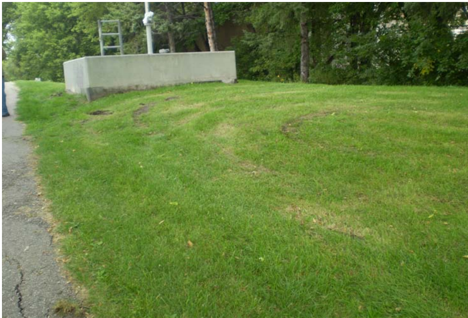
Photo 22- Elmwood Park: Ruts from vehicles by concrete chamber.
