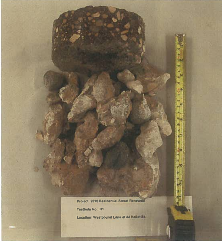
Photo 9: Test Hole H1: 44 Hallet St., Westbound Lane, 35 m E of W sidewalk at Rover Ave., 1.9m S of N curb
