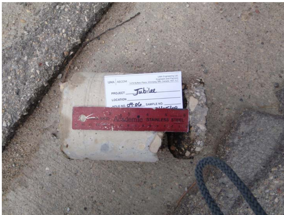
Photo 06: Pavement core at the location of TH 09-06
