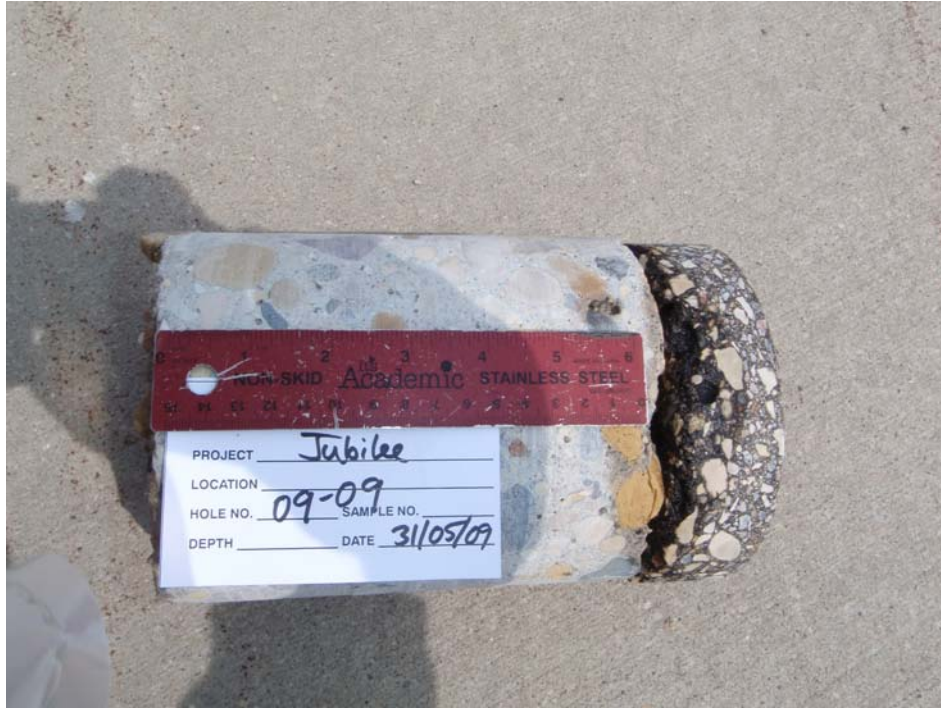
Photo 09: Pavement core at the location of TH 09-09
