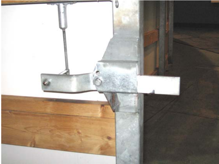
VA 5: Player's Gate Latch Detail
