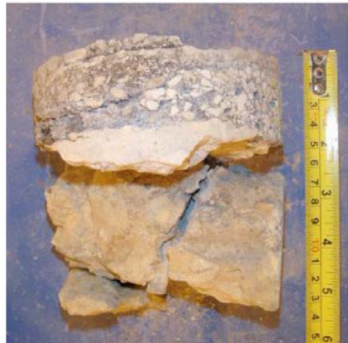
Core sample from Testhole TH2
