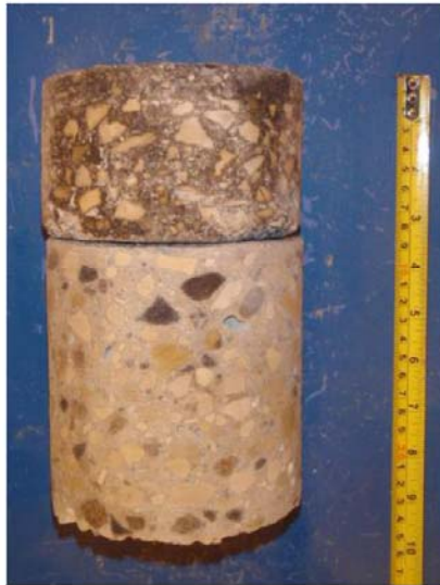
Core sample from Testhole TH5
