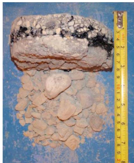
Core sample from Testhole TH3
