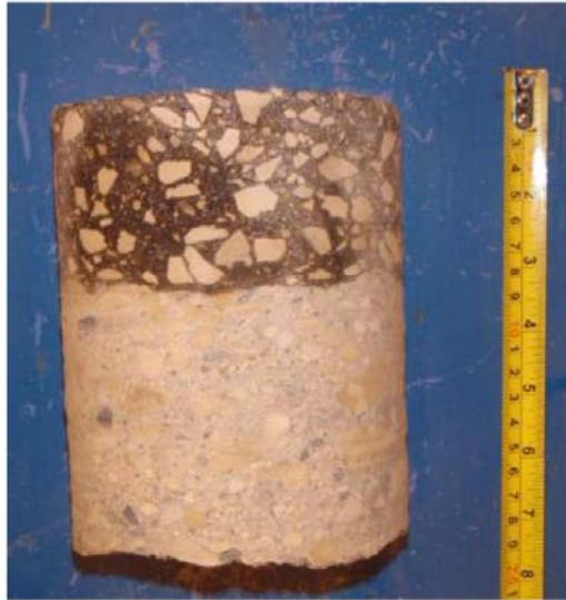
Core sample from Testhole TH6
