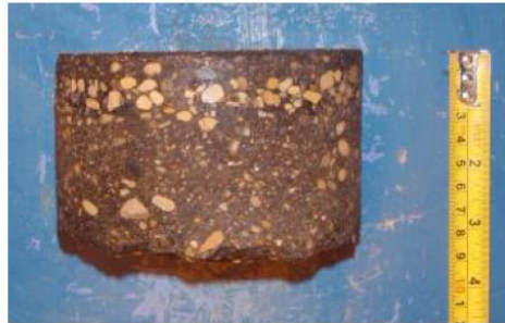
Core sample from Testhole TH1
