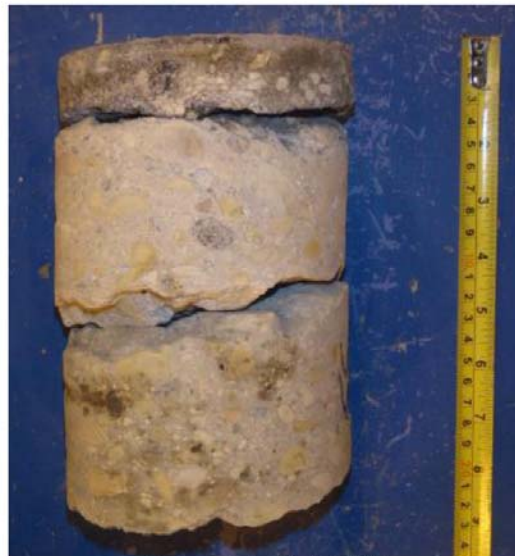
Core sample from Testhole TH3
