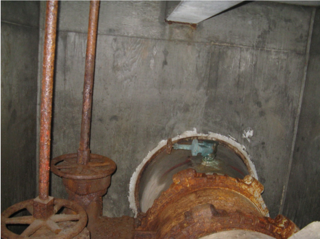
South and East Pipe and Valve Condition (3)
