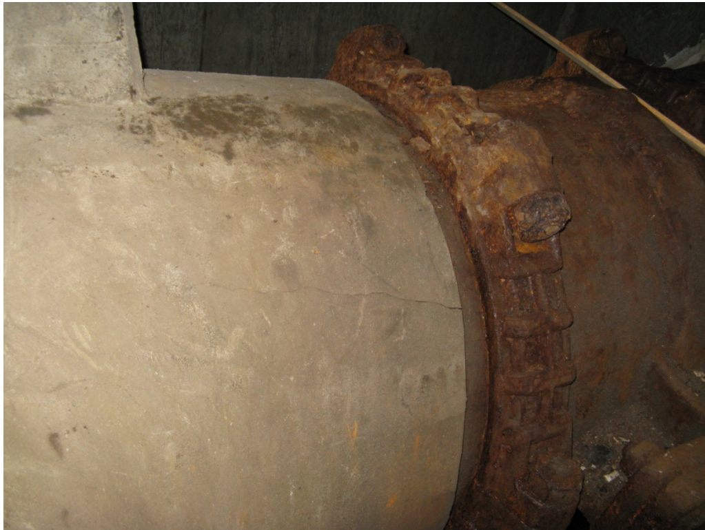
North Pipe and Valve Condition
