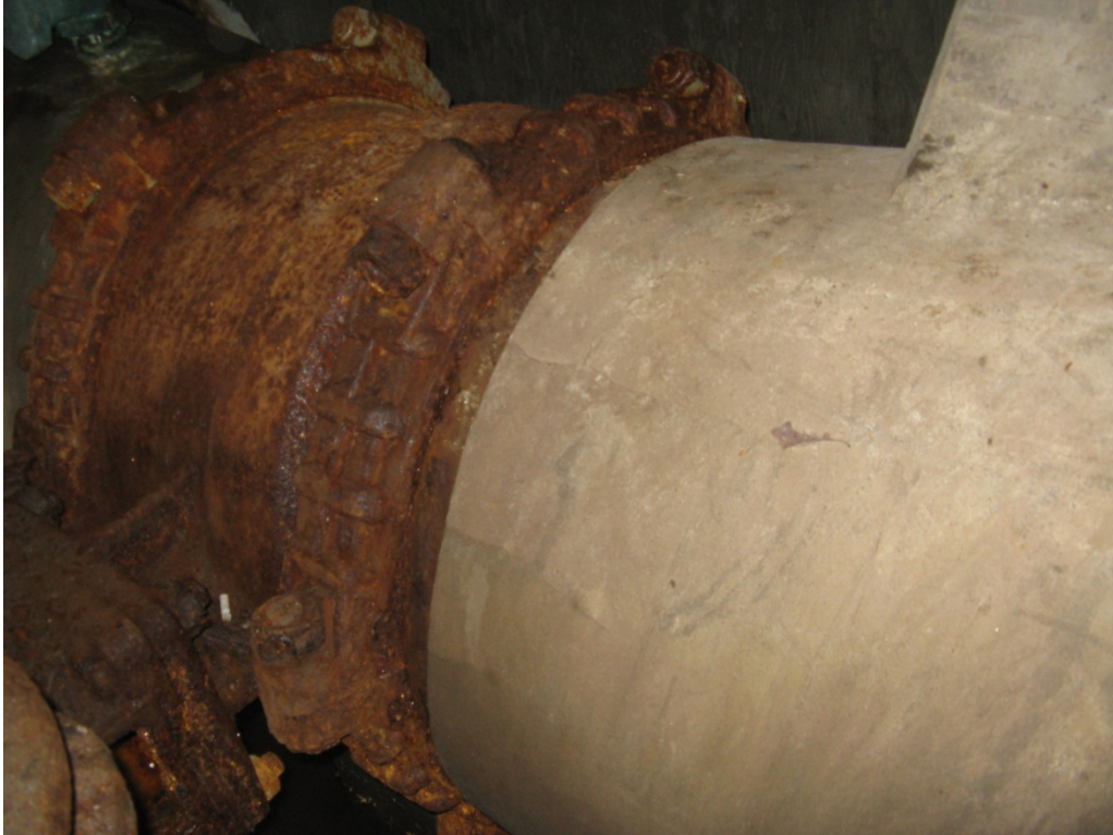
South Pipe and Valve Condition
