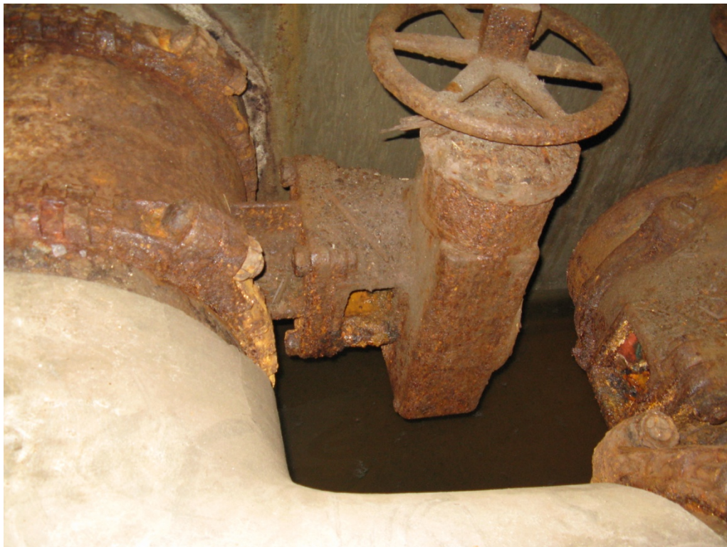
South and East Pipe and Valve Condition (1)
