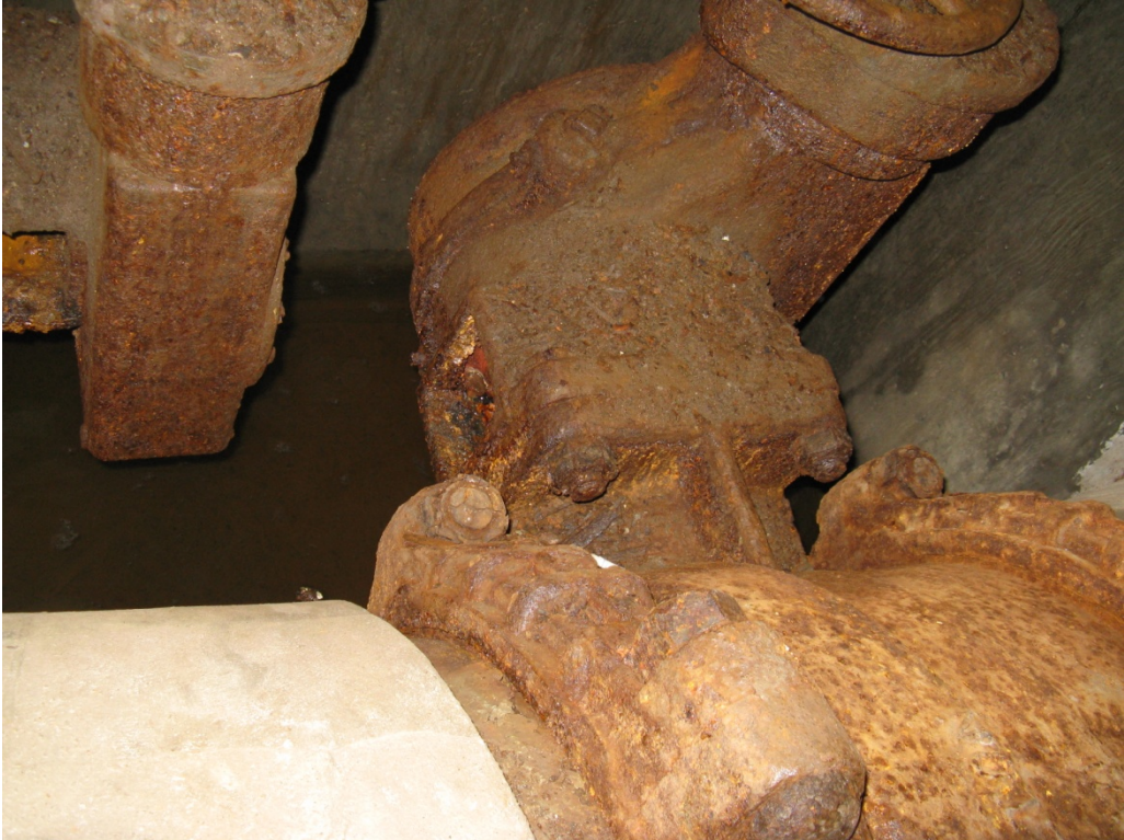
South and East Pipe and Valve Condition (2)
