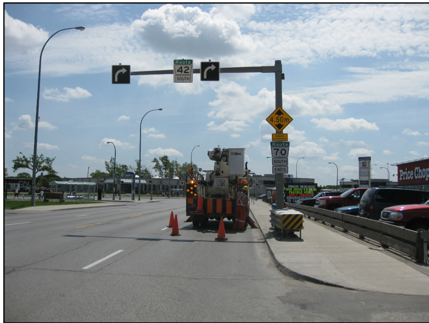
STRUCTURE ELEVATION – LOOKING SOUTH
