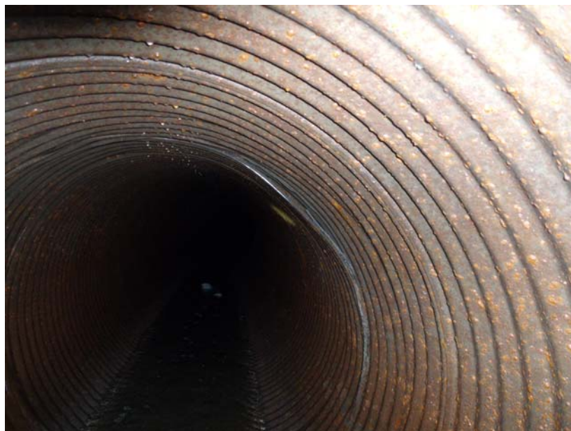
Figure 7: Open Joint 2 – Looking down stream
