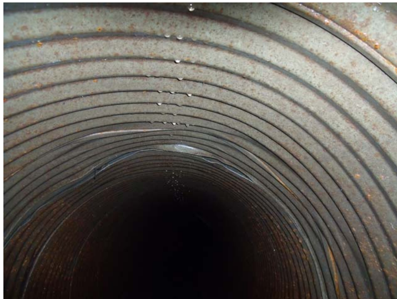
Figure 5: Open joint 1 - Looking downstream
