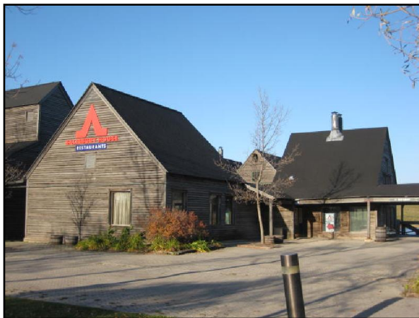
Exterior View - Harbourview Recreation Complex
