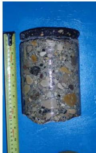
Core sample from Testhole TH4
