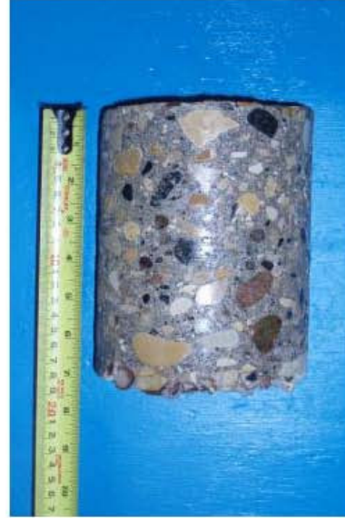
Core sample from Testhole TH2
