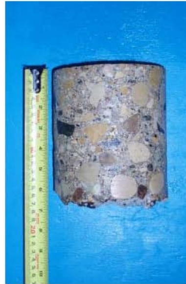
Core sample from Testhole TH2
