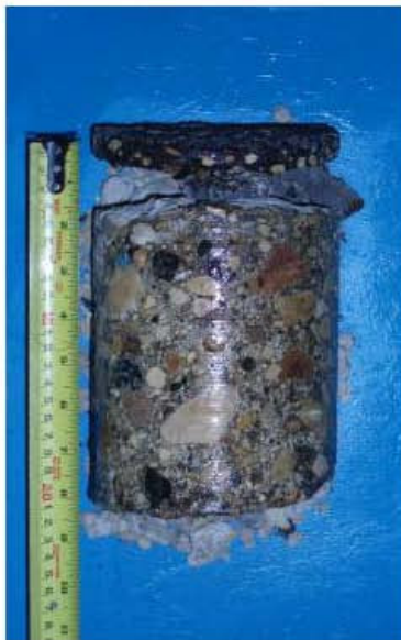
Core sample from Testhole TH3
