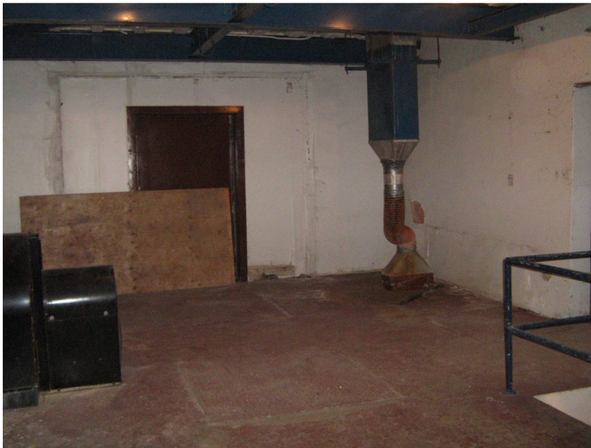
Figure 1 : Mechanical Room - South-East View
