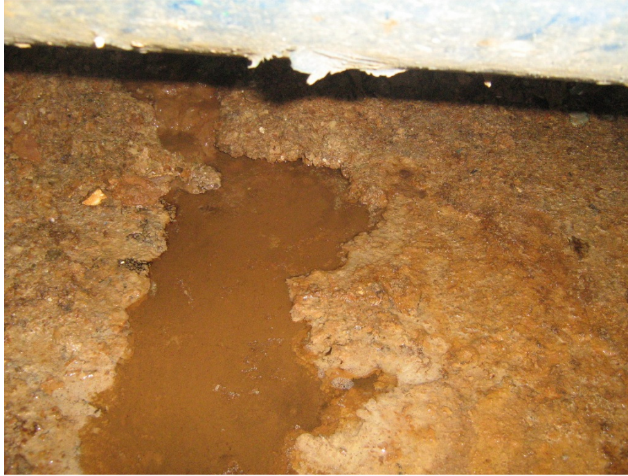
Figure 10 : Pump Room Floor
