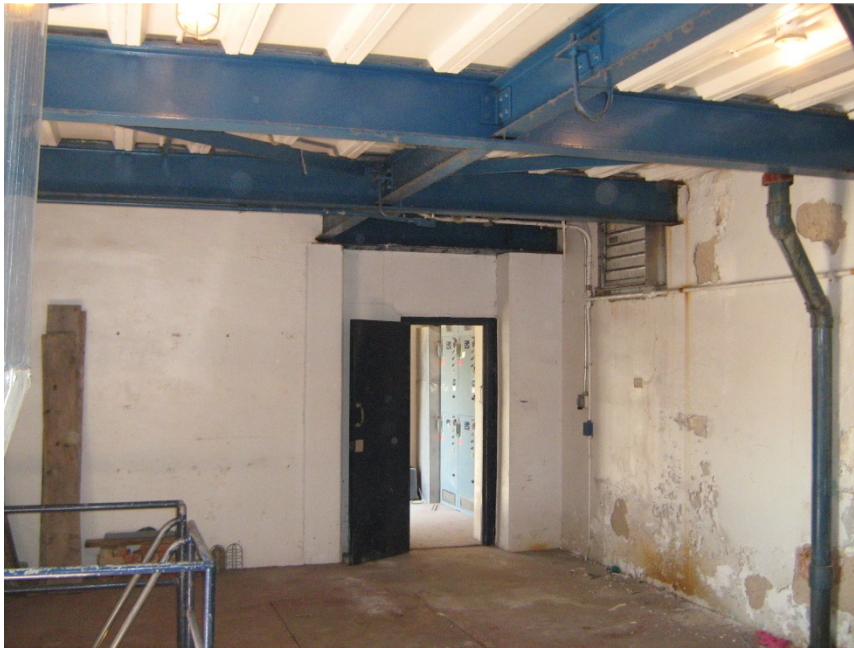
Figure 2 : Mechanical Room - North-West View
