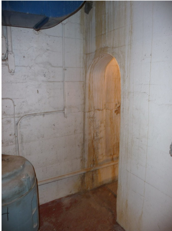
Figure 8 : Motor Room Walls
