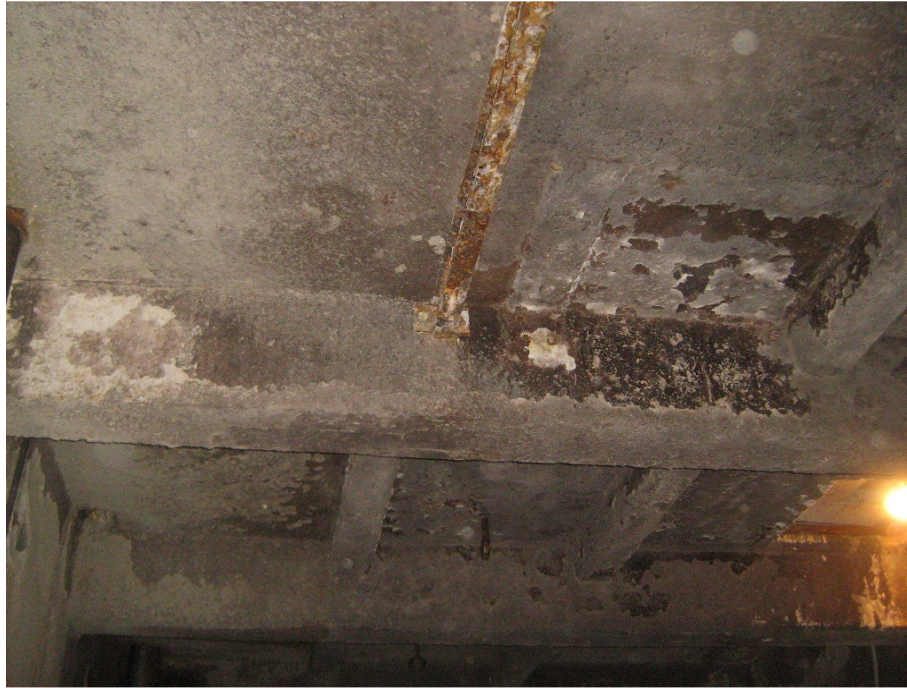
Figure 7 : Comminutor Chamber Steel Beam
