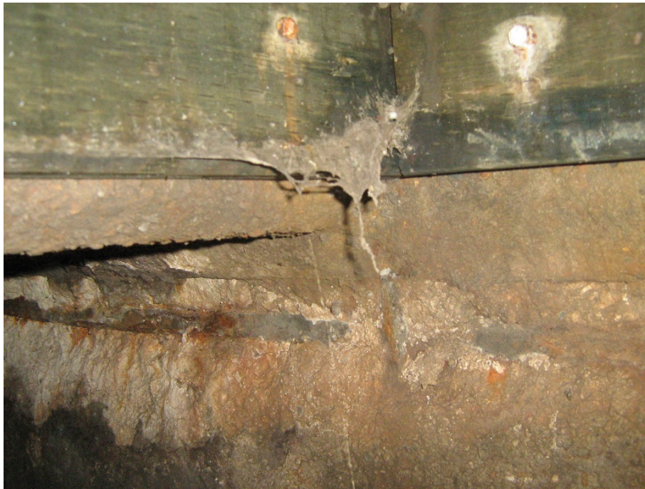
Figure 6 : Comminutor Chamber Stairway Opening
