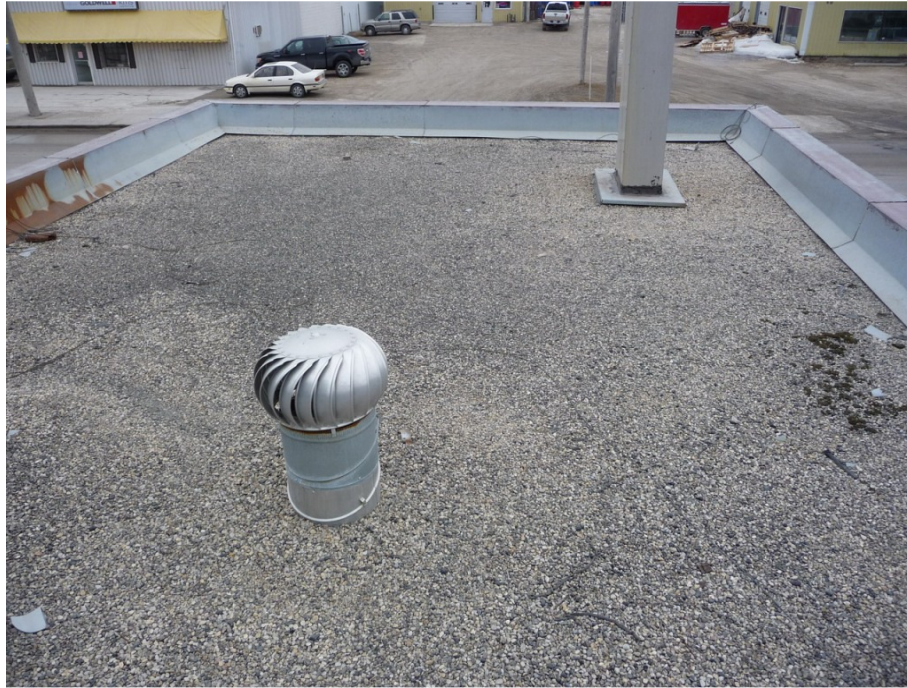
Figure 13 : Montcalm Pumping Station Roof
