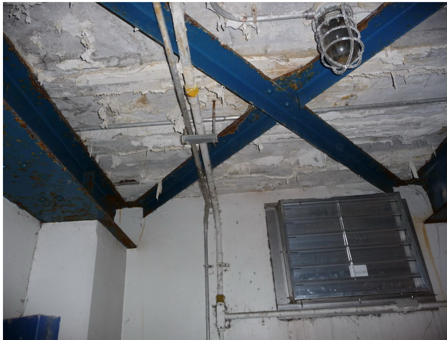
Figure 3 : Mechanical Room Ceiling
