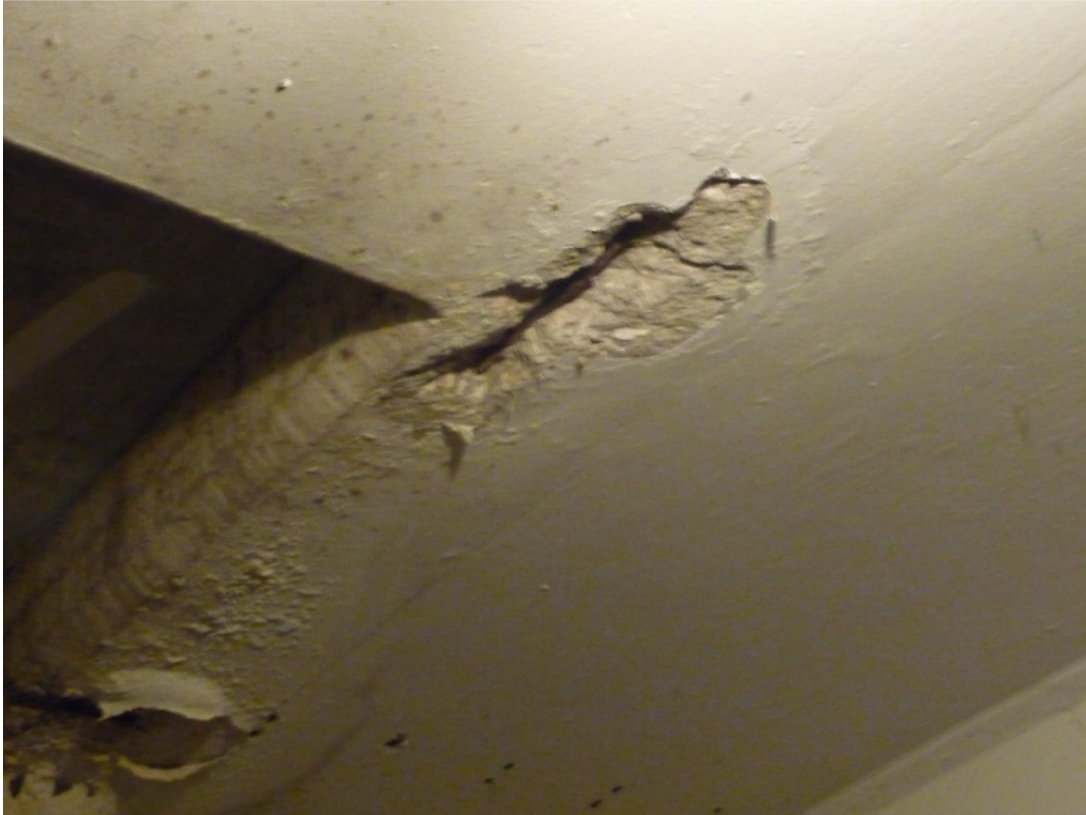
Figure 5 : Comminutor Motor Room Ceiling Hatch
