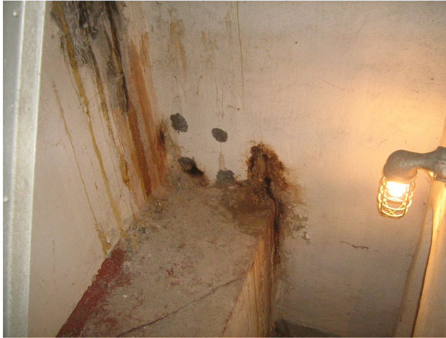
Figure 12 : Stairwell Leaks
