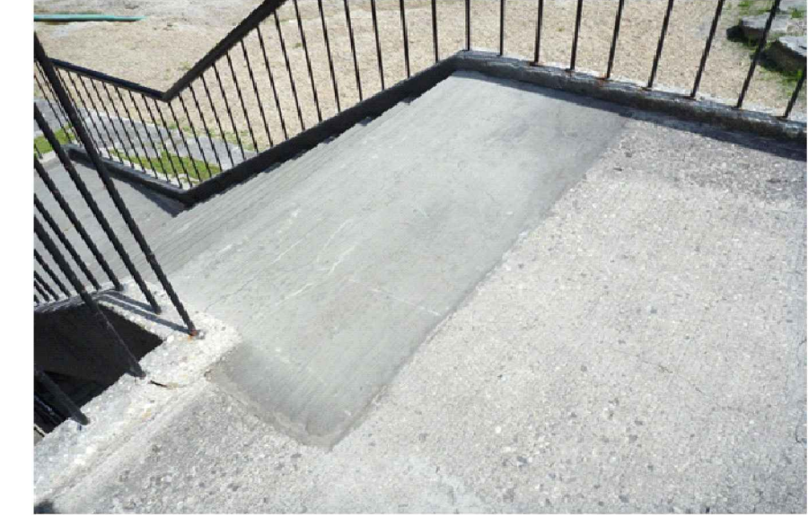
PHOTO #5: TOP SURFACE OF LANDING SHOWING SKIM COAT REPAIR.
