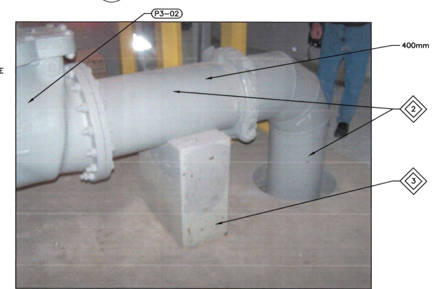
6 P3 DISCHARGE PIPING - LEVEL 200 M1
