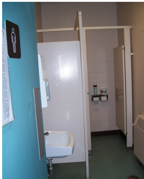
Figure 20.18: Existing Men's Washroom - Main Floor
