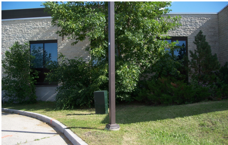
Figure 20.25: Exterior - North Side of New Addition
