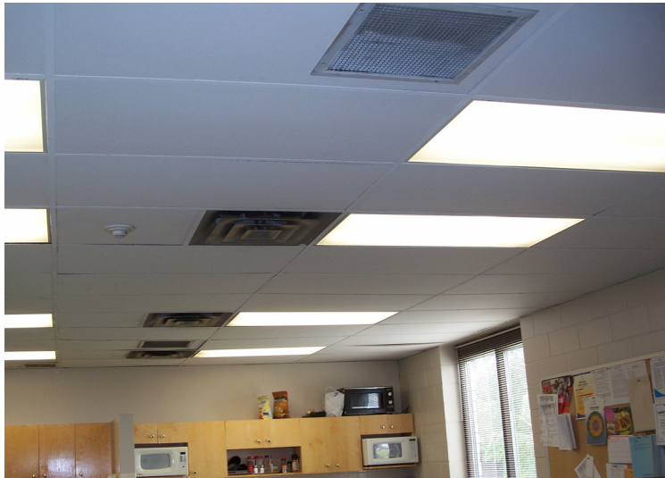
Figure 20.9: Lunch Room / Classroom - Ceiling Panels and Lighting
