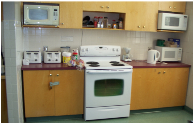
Figure 20.8: Lunch Room / Classroom - Kitchen Appliances
