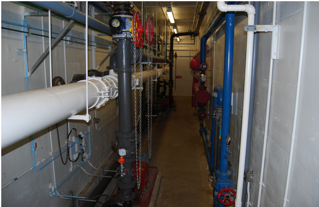
Figure 22.16: Gallery No. 4 (influent end of PST No. 1 & 2) facing north. Area ID #15.
