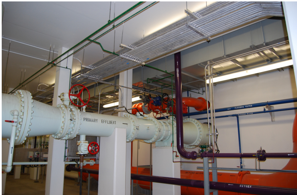
Figure 22.20: Gallery No. 5 (PST No. 3 effluent end) facing south. Area ID #17.
