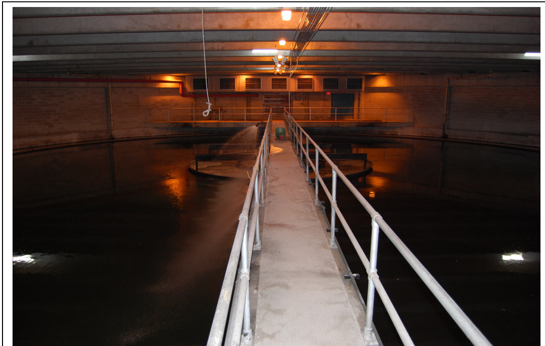
Figure 22.29: Secondary Clarifier No. 1 facing north. Area ID #26.
