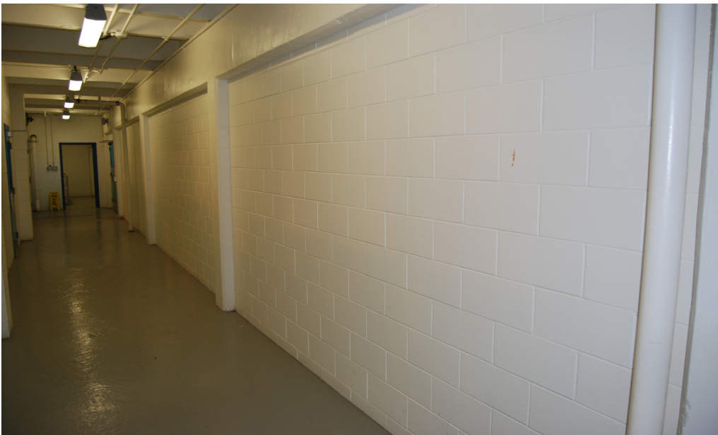
Figure 22.4: Hallway west of Grit Room facing south. Area ID #8.
