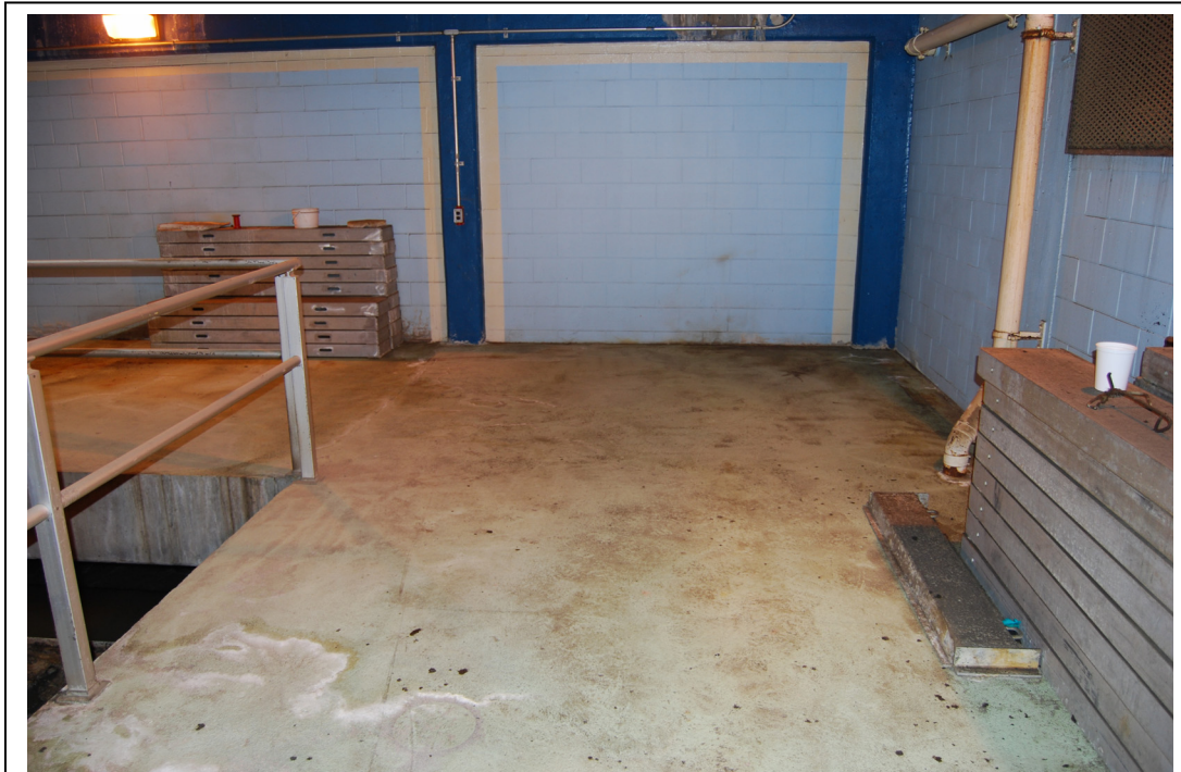
Figure 22.6: Grit Room southeast corner. Area ID #10.
