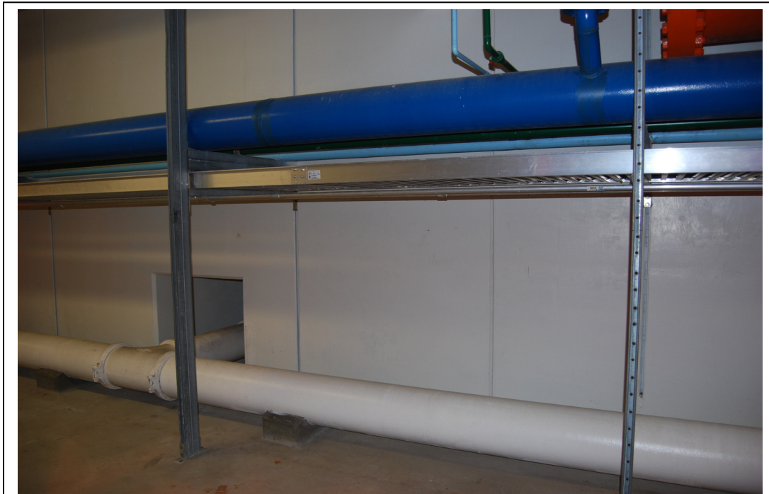
Figure 22.30: Gallery No. 3 facing north at Secondary Clarifier No. 3. Area ID #27.
