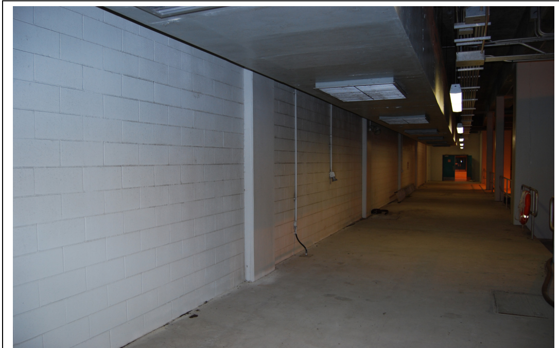
Figure 22.31: Secondary Clarifier No. 3 main floor facing north. Area ID #28.
