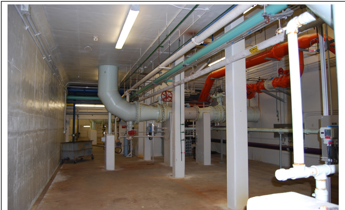
Figure 22.18: Gallery No. 5 (PST No. 1 & 2 effluent end) facing south. Area ID #17.
