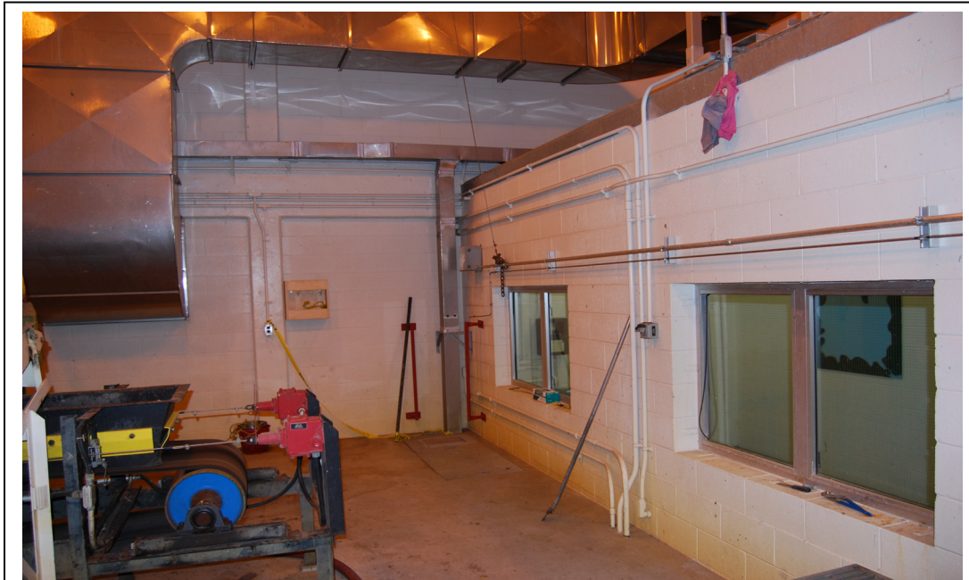
Figure 22.3: Screen Room southwest corner. Area ID #7.
