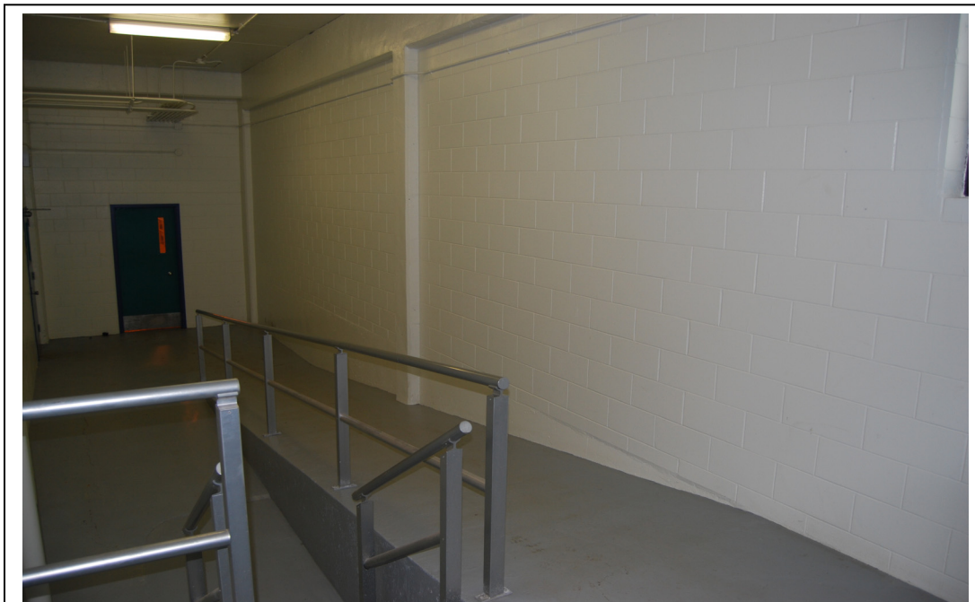
Figure 22.11: Hallway from Grit Room to PST facing west. Area ID #12.
