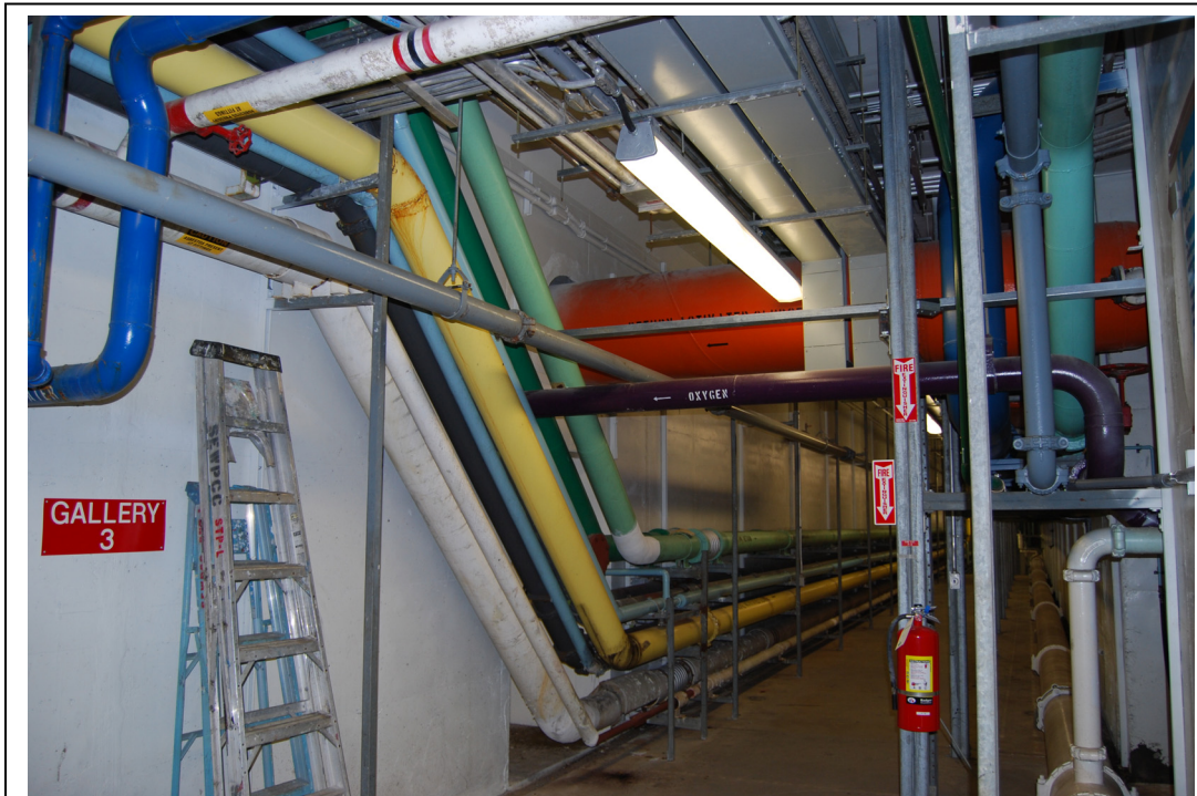
Figure 22.21: Gallery No. 3 at entrance to Gallery No. 5. Area ID #17.
