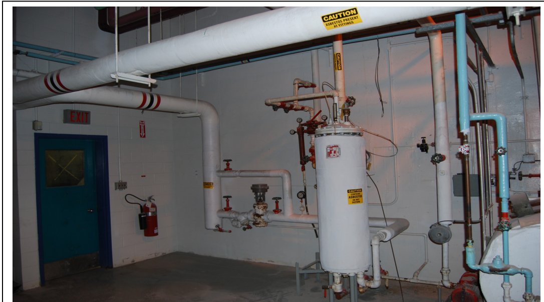
Figure 22.10: Boiler Room southeast corner. Area ID #11.
