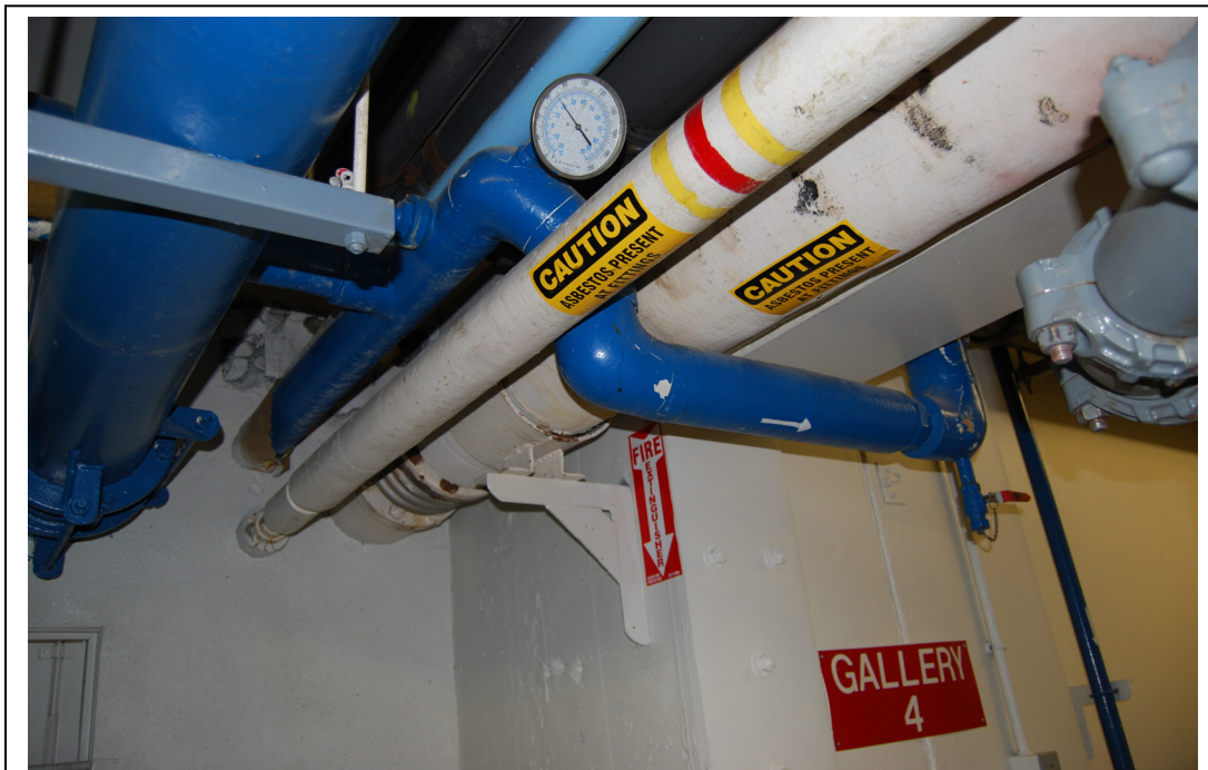
Figure 22.13: Gallery No.3 at entrance to Gallery No. 4 facing east. Area ID #14.
