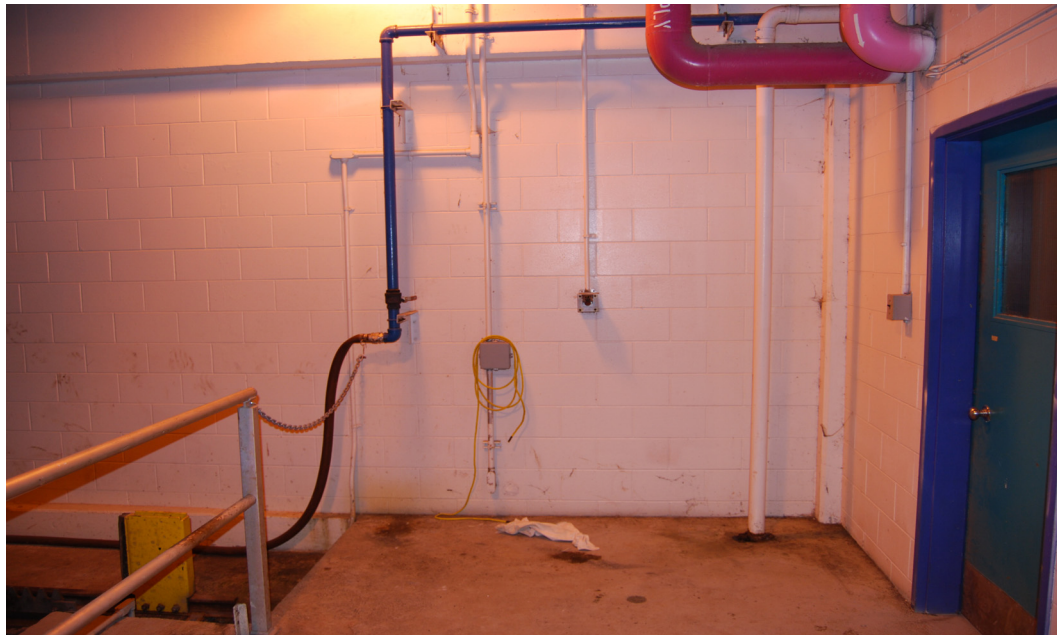
Figure 22.17: Influent end of PST No. 2 & 3 facing north wall. Area ID #16.
