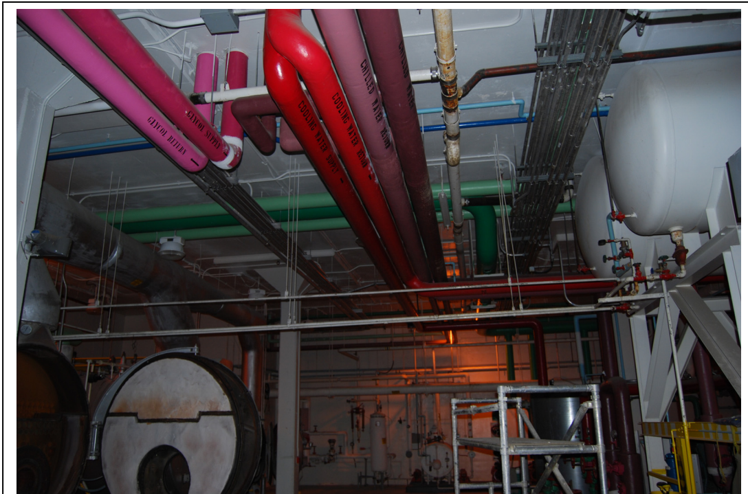
Figure 22.9: Boiler Room facing south. Area ID #11.
