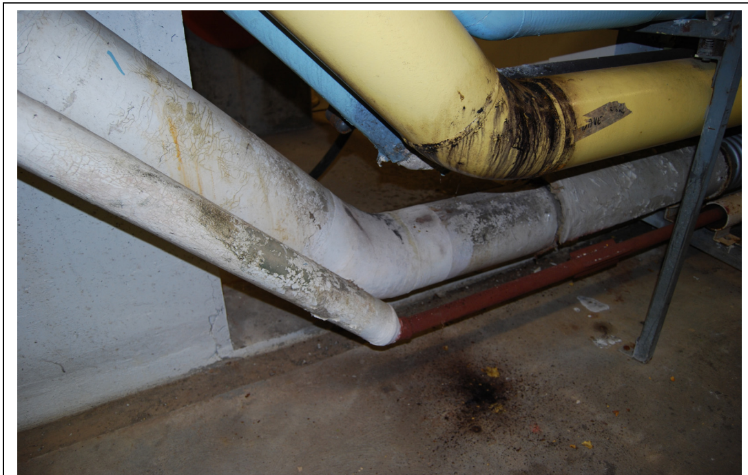
Figure 22.22: Gallery No. 3 at entrance to Gallery No. 5. Area ID #17.
