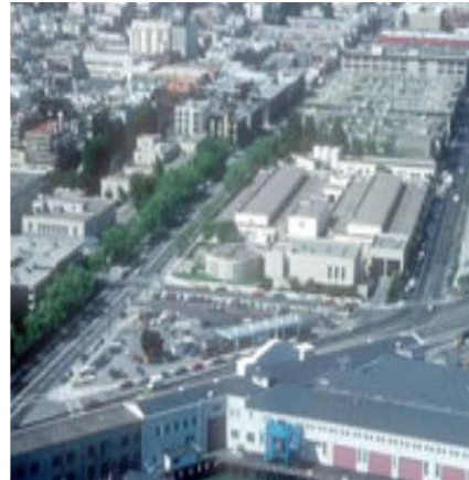
North Point Facility
