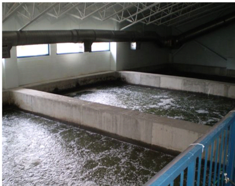
Figure 7.2: Covered Building in a BAF plant at Boisbriand, Quebec (Source: John Meunier)
