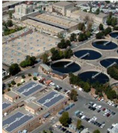
Southeast Water Pollution Control Plant
