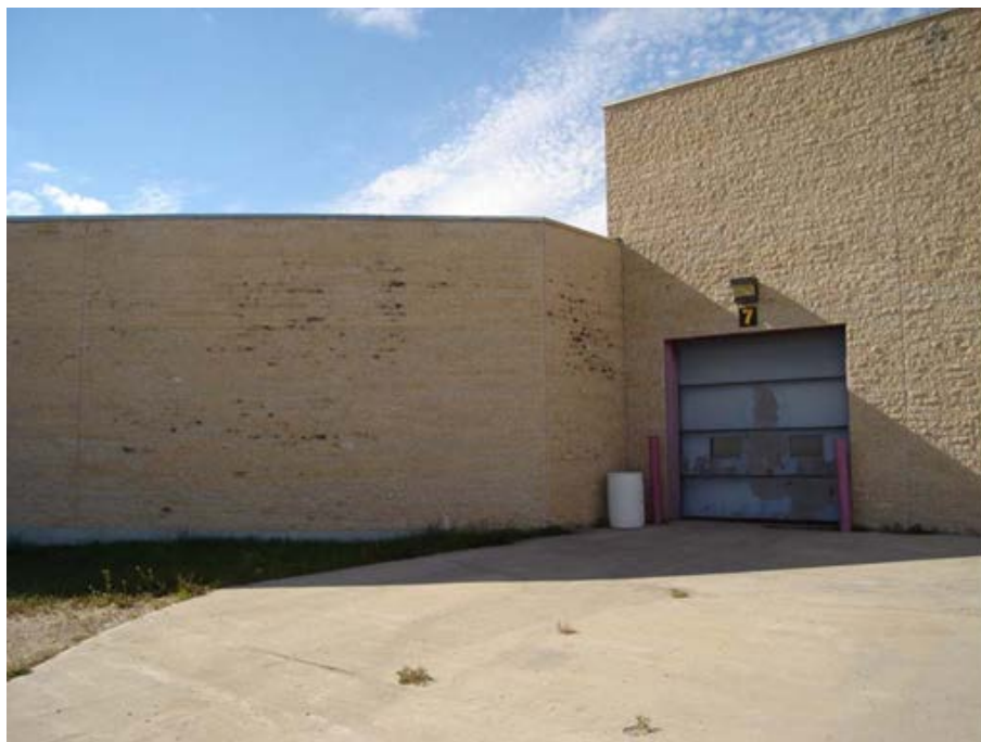
Photo 1.3-26 – SLUDGE THICKENING AND SLUDGE TRUCK BAY STRUCTURE Southwest Corner of Sludge Thickening
