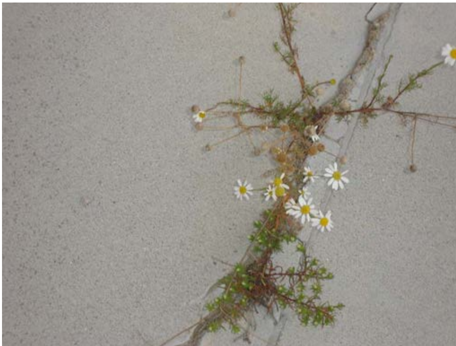
Photo 1.3-24 – OXYGEN REACTORS NOS. 3 AND 4 STRUCTURE Typical Vegetation Growth – Roof Top
