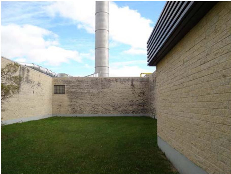
Photo 1.3-20 – PRIMARY CLARIFIER NOS. 1 AND 2 STRUCTURE Link to Grit Building – North Elevation – East End In June 2009, cleaning work was undertaken under Work Order 09042880. Additional cleaning is required and Work Order 1004092 was issued in May 2010. The cleaning work is yet to be completed.
